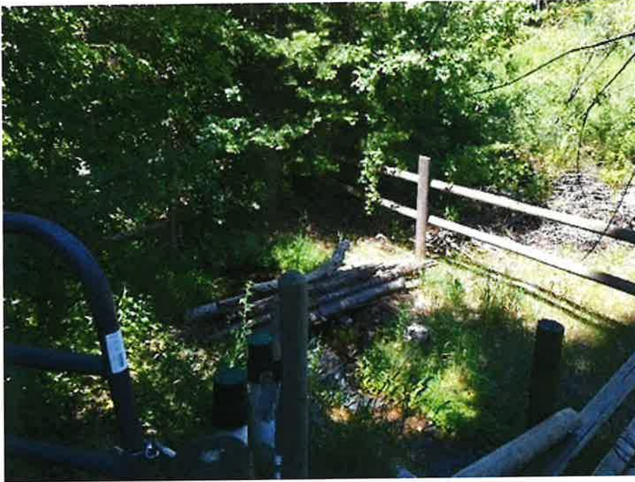
Overall point of diversion. Controlling works are in place and can be accessed through the vertical PVC pipes just beyond the gate.
