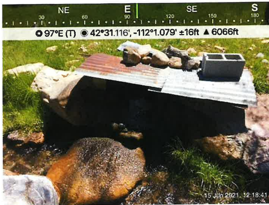
Point of re-diversion into the stream channel.
