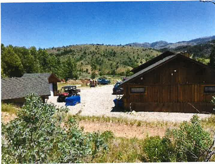
Cabin and out buildings where power is used.
