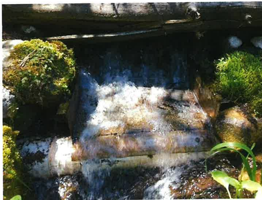
Point of diversion with screen.
