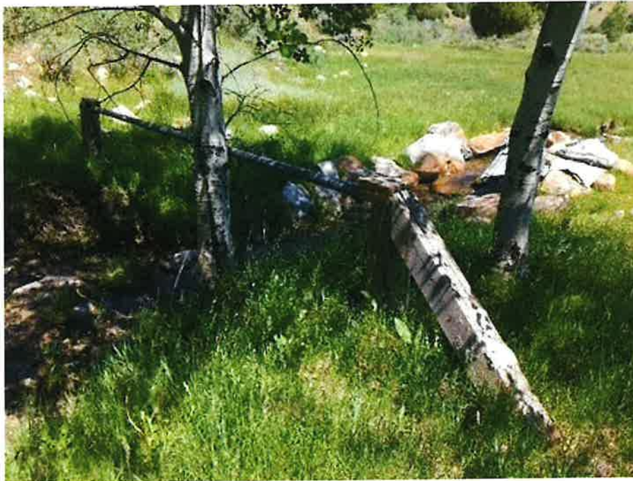
Overall photo of the re-diversion. A power line was constructed going over the stream.
