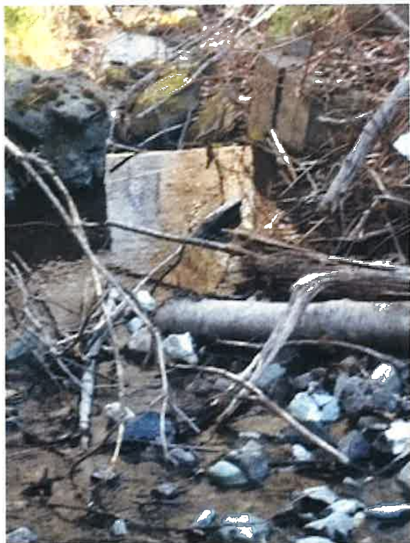
Diversion in Shingle Creek. 45°21'50.55"N, 116°24'11.96"W
