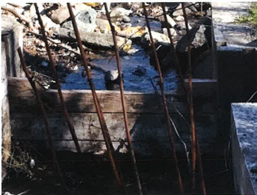
Diversion in Shingle Creek. With board in place, flow diverts back to creek. 45°21'50.55"N, 116°24'11.96"W
