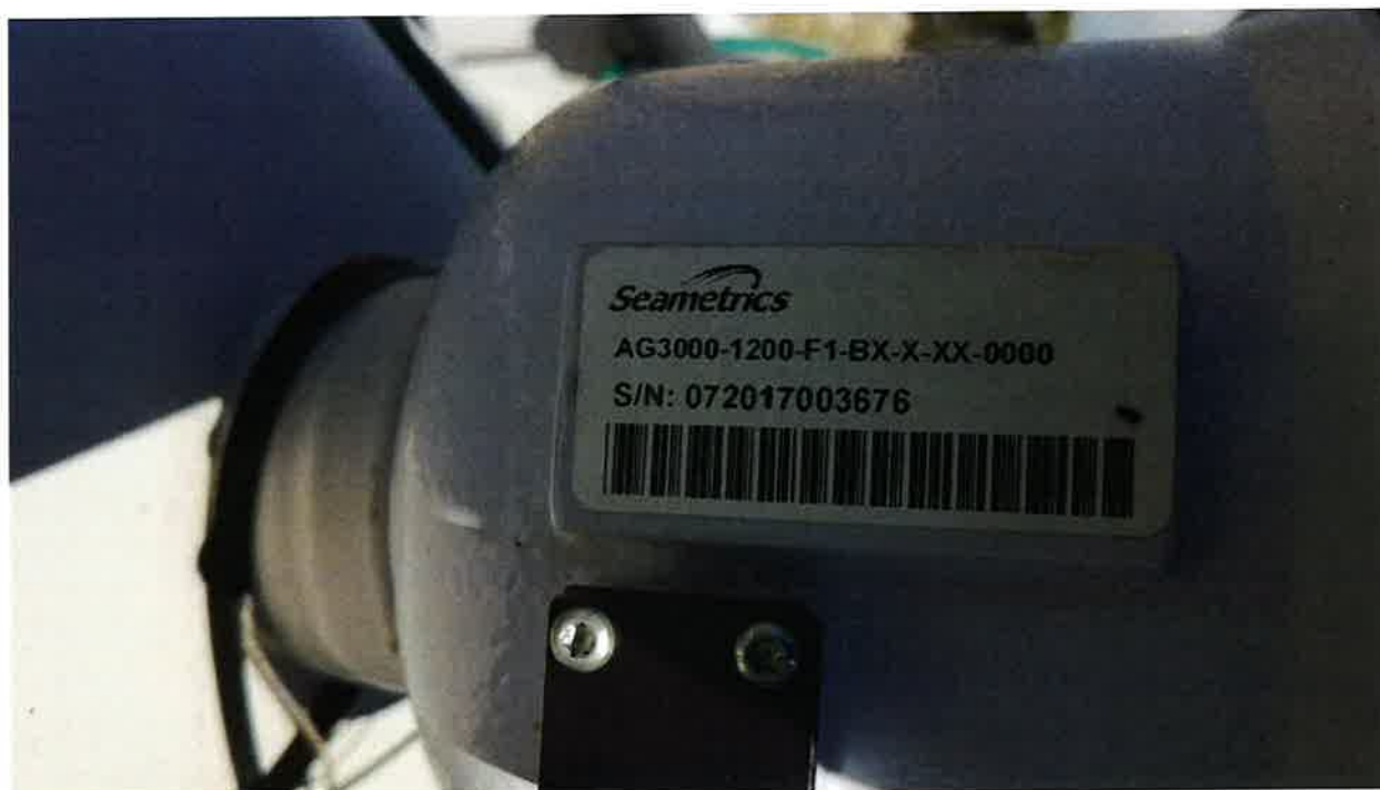
Figure 19: Well 2 flow meter information
