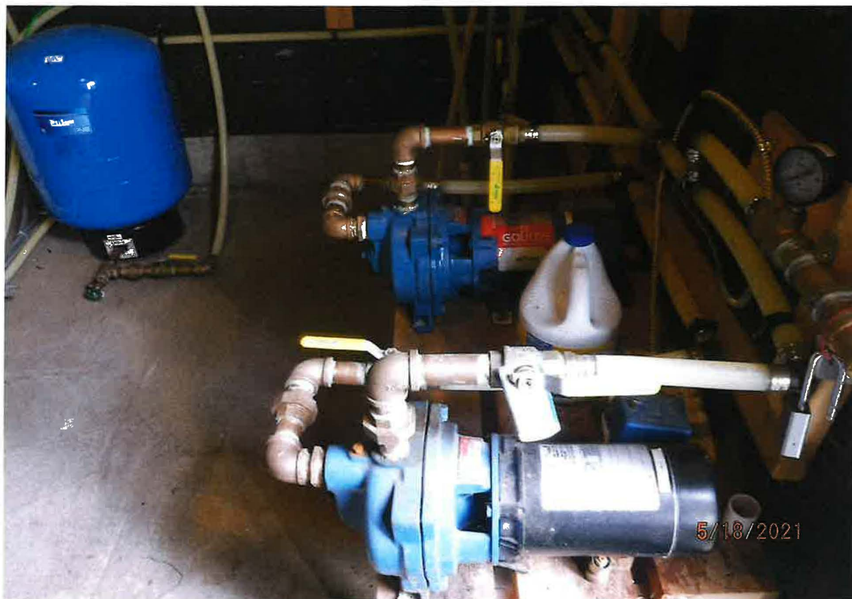
2EA ONE HP DISTRIIBUTION PUMPS FROM RESERVOIR SERVICES SYSTEM
