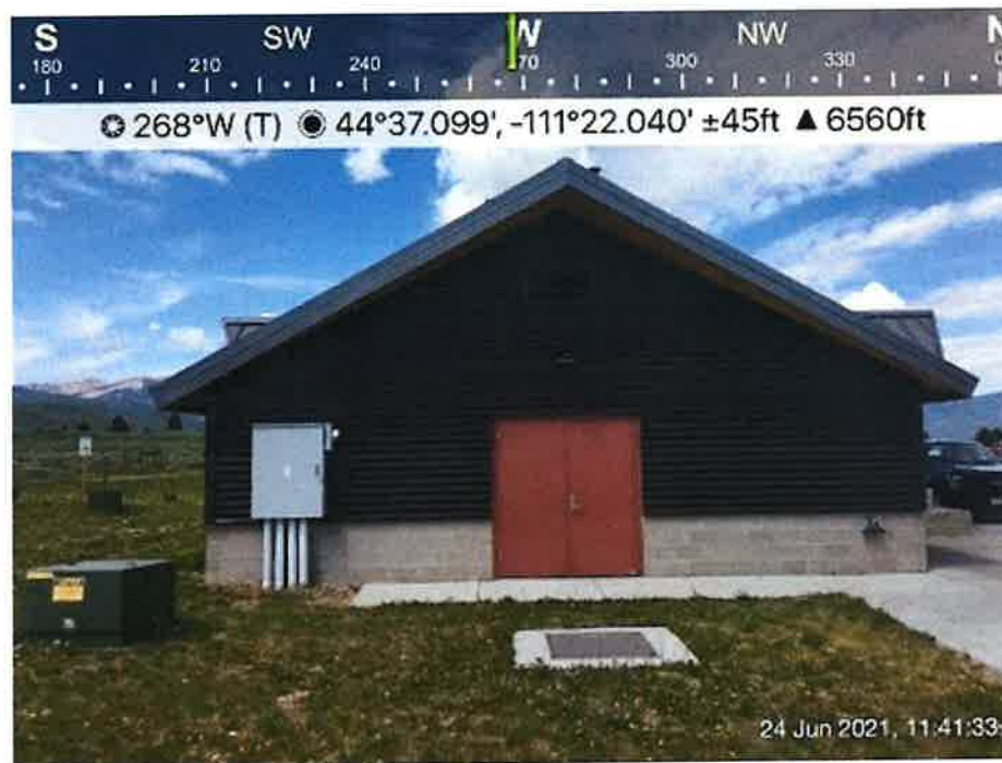
Utility and control room for the Shower Building and is the location for the flow meter for Well No. 2. Located on the east end of the building.
