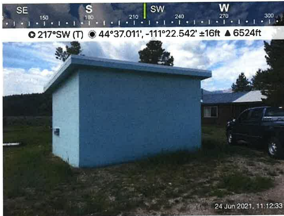
Well house for Well No. 1.
