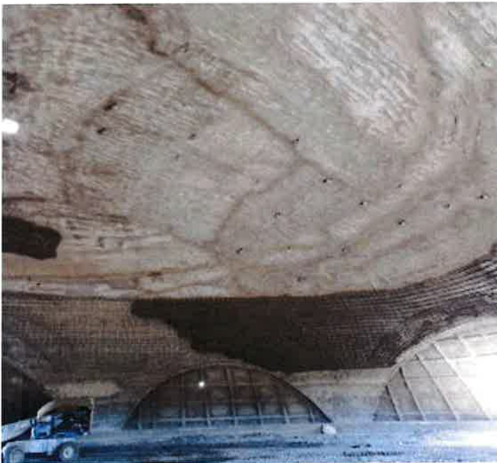
Fig. 1: Reinforcing bars and shotcrete are integral parts of the dome construction process
