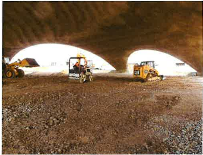
Fig. 3: Openings are made to the dome shell, which allow light to enter the completed office
