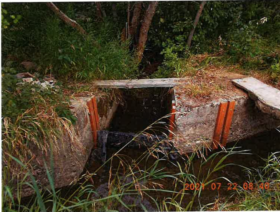
52 53 Photo 2752. Structure at Location B. 54
