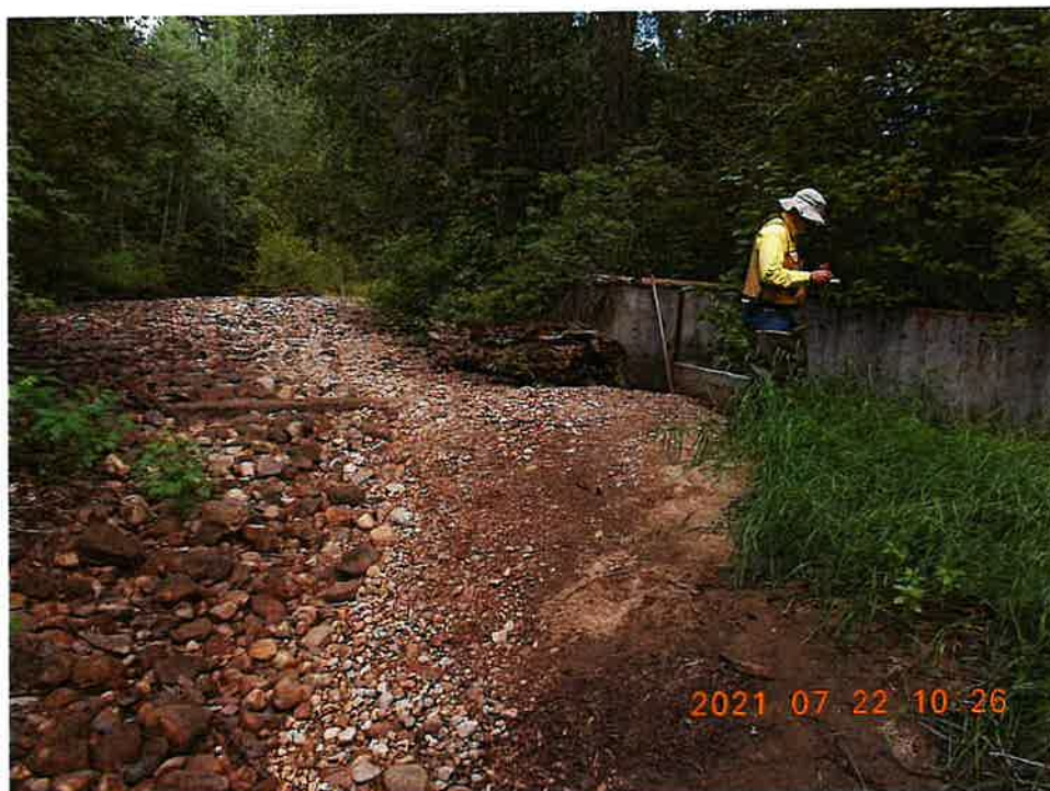
Photo 2779. North Leigh Creek at Hubbard Diversion.
