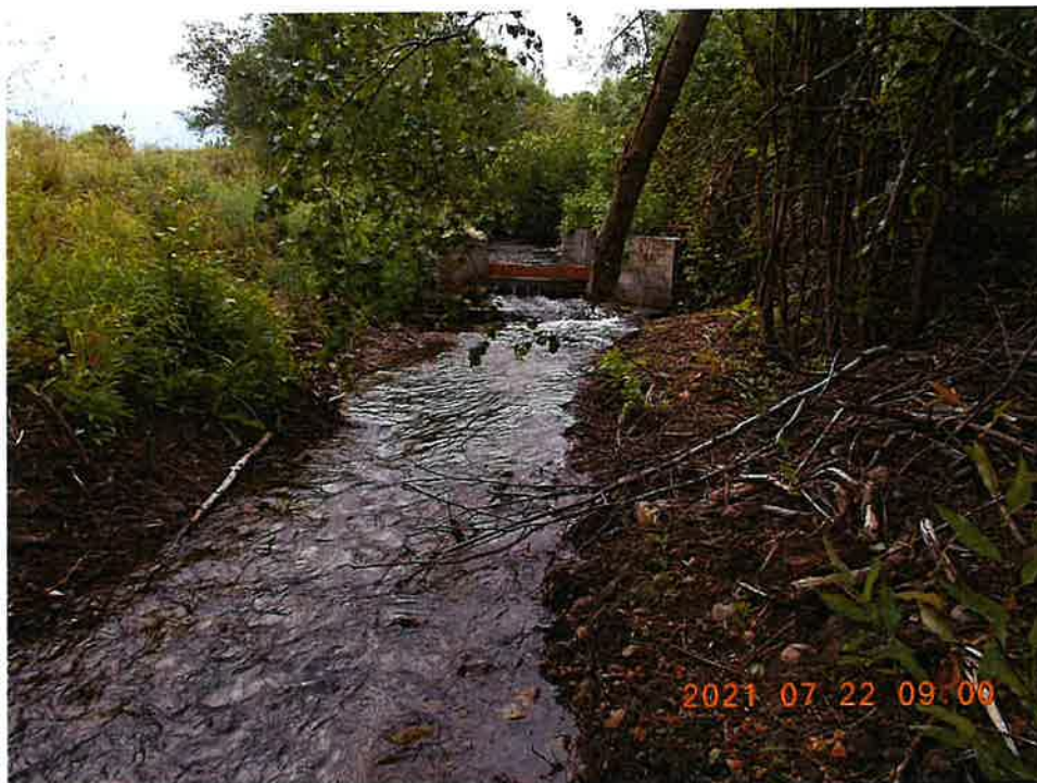
27 28 Photo 2763. Looking upstream on the Grouse Creek Ditch toward the structure at Point 29 A on the Figures. 30
