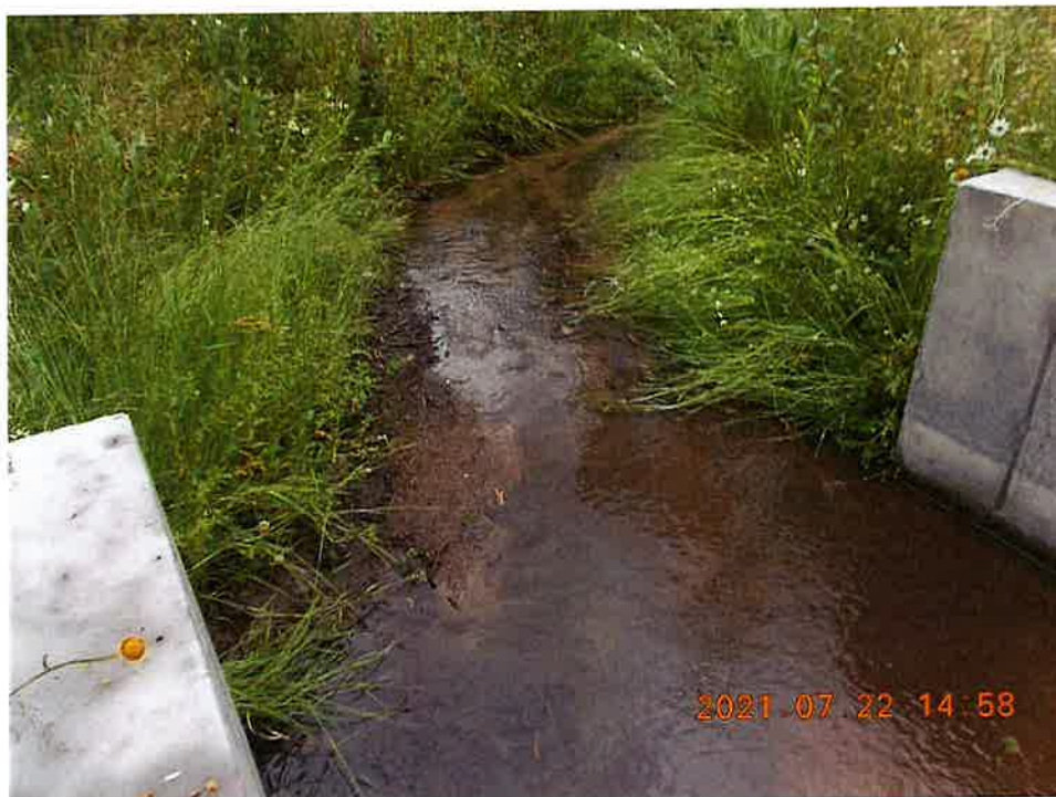
182 183 Photo 2812. Looking downstream from the south outlet of the splitter structure. This 184 outlet supplies a lateral that turns and heads due west. 185
