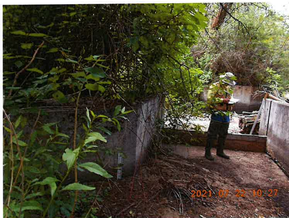
Photo 2785. Looking upstream at the diversion structure from the head of Hubbard Ditch.
