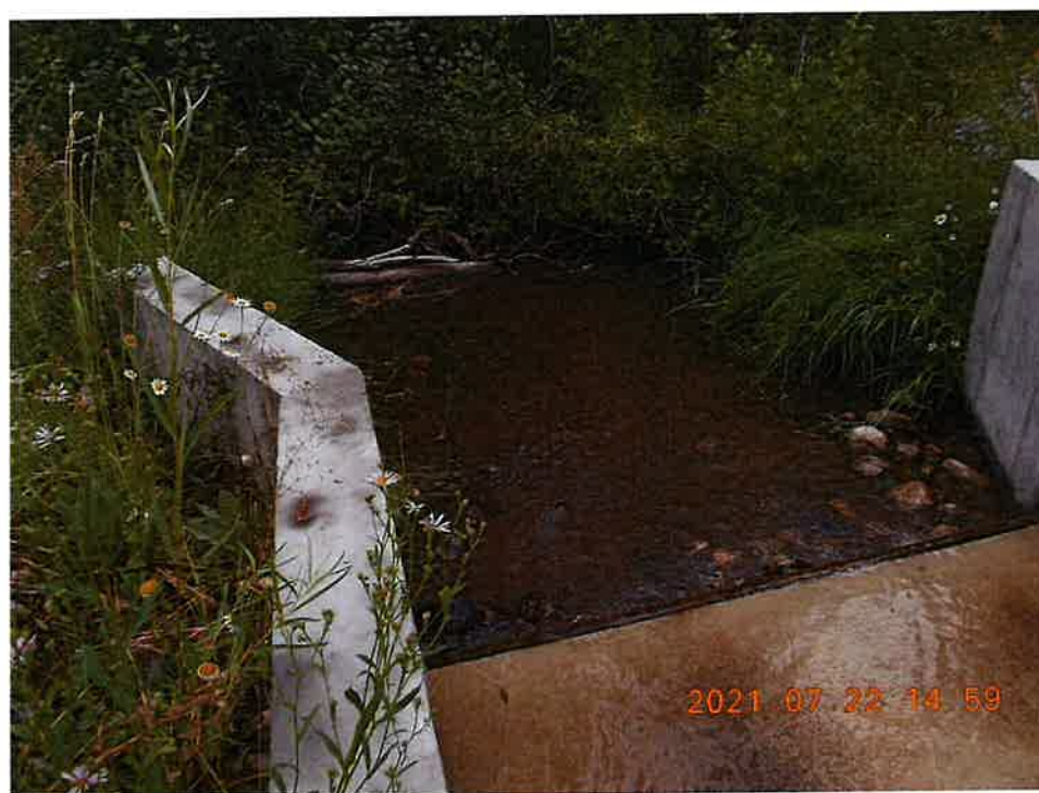
186 187 Photo 2815. Looking downstream on the west (Hubbard Ditch) outlet of the splitter 188 structure.
