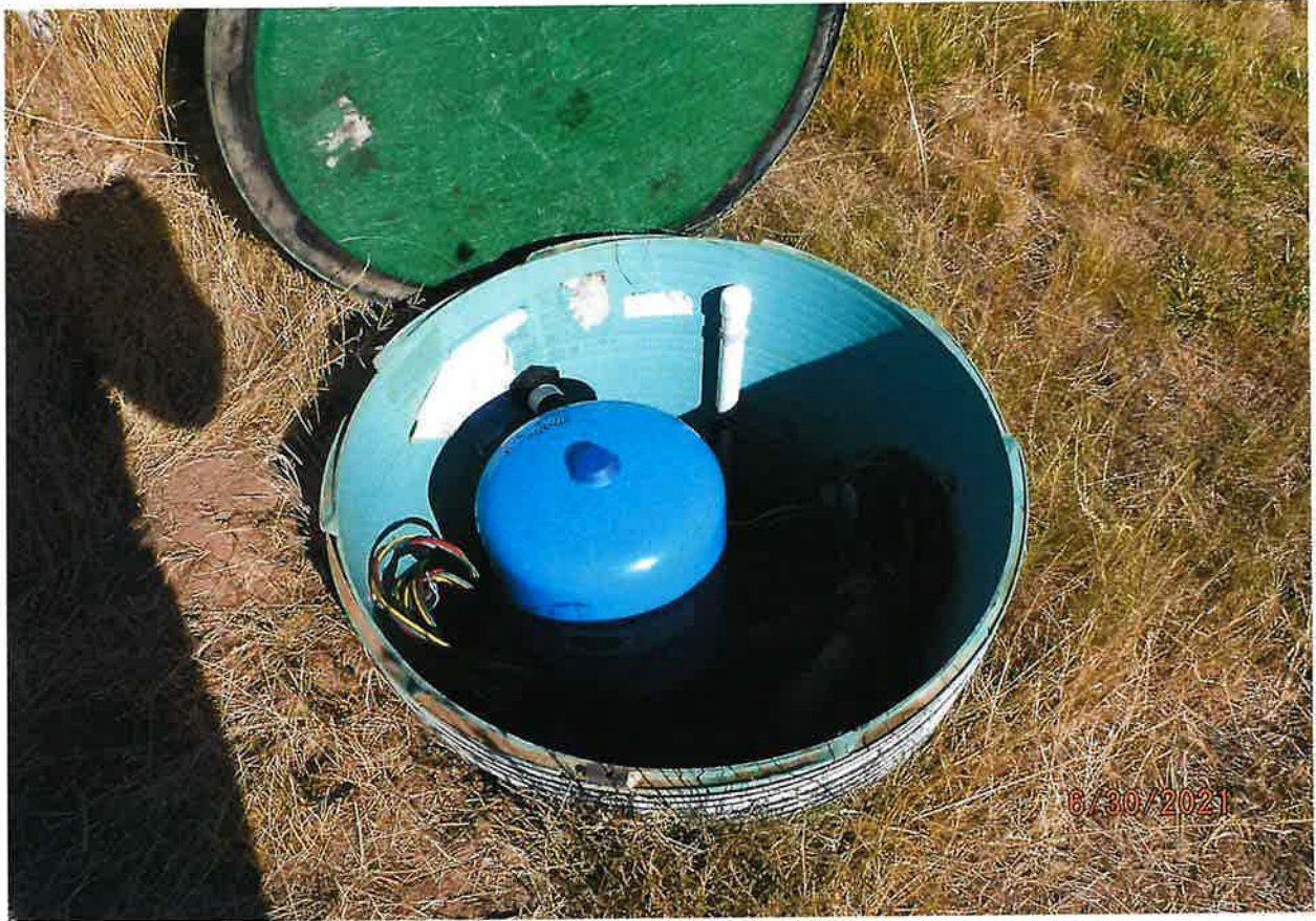
2,000 GALLON STORAGE RESERVOIR WITH PRESSURE POT
