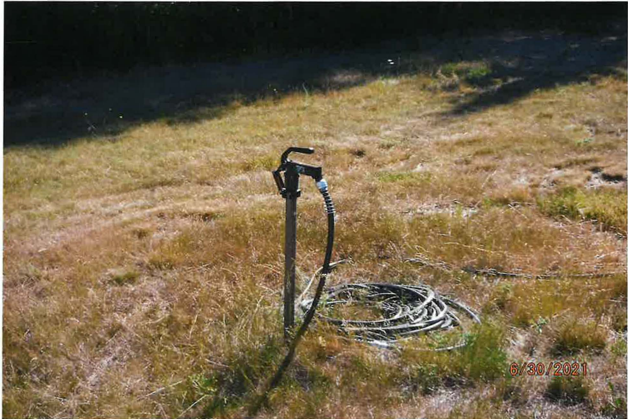
IRRIGATION BY PRESSURIZED SPRINKLERS, FROST FREE HYDRANT TO HOSE/SPRINKLER, & SMALL EMMITTERS AND SOAKER HOSES.
