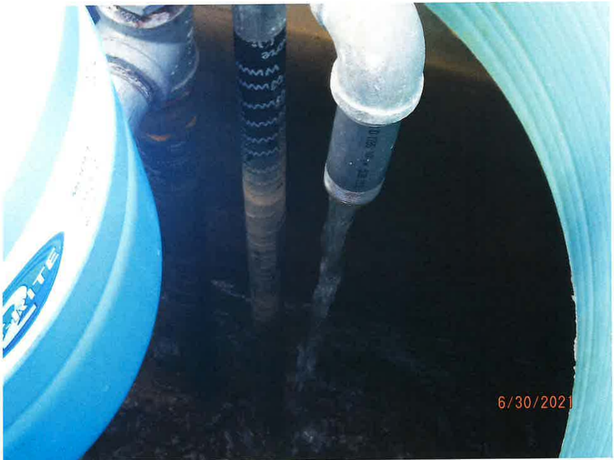
2,000 GALLON STORAGE RESERVOIR WITH PRESSURE POT
