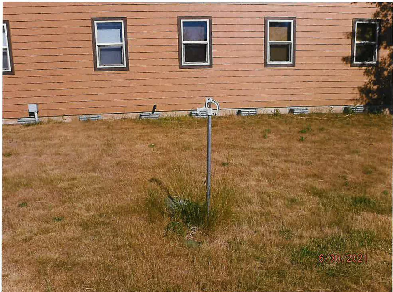
IRRIGATION BY PRESSURIZED SPRINKLERS, FROST FREE HYDRANT TO HOSE/SPRINKLER, & SMALL EMMITTERS AND SOAKER HOSES.
