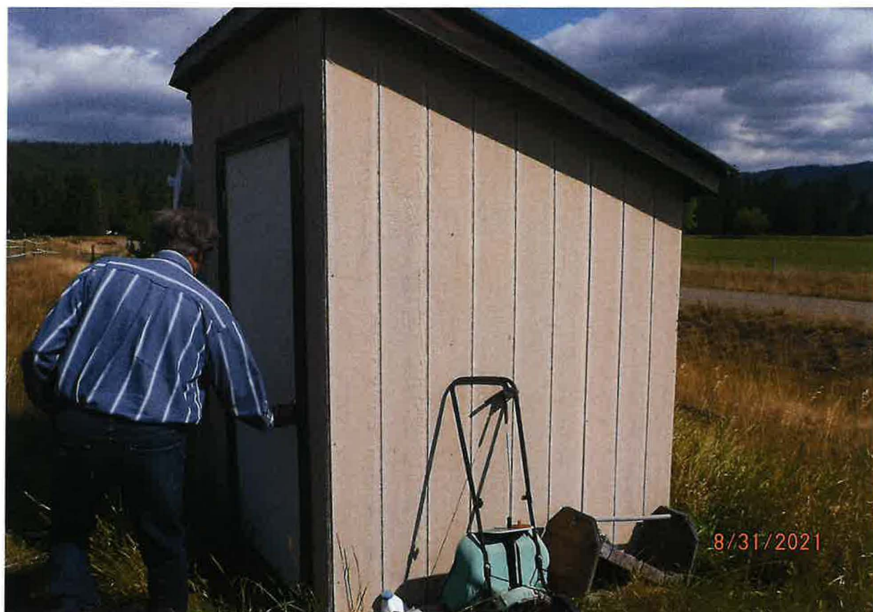
PUMP STATION STRUCTURE
