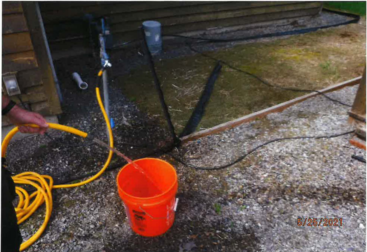
FLOW MEASUREMENT FROM FROST FREE HYDRANT – GRAVITY FLOW FED FROM 2EA SPRINGS
