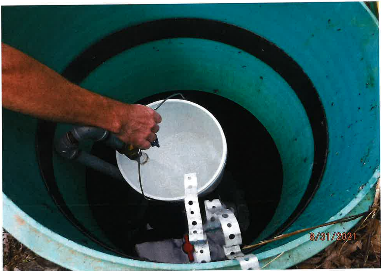
5 GAL BUCKET TEST MEASURED FLOW FROM 1 ST STORAGE INFLOW PIPE FROM POD
