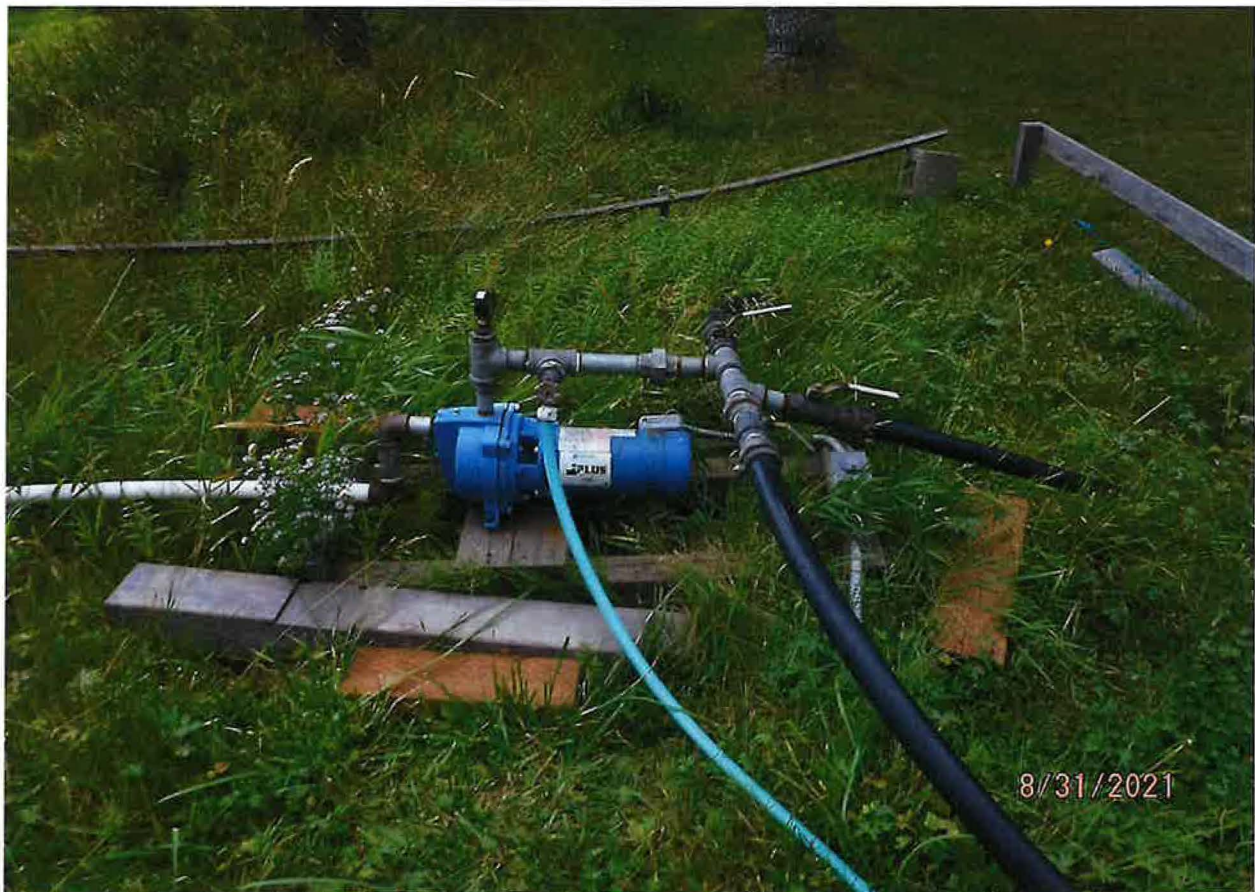
DIVERTING WORKS – 1 HP GOULDS PUMP
