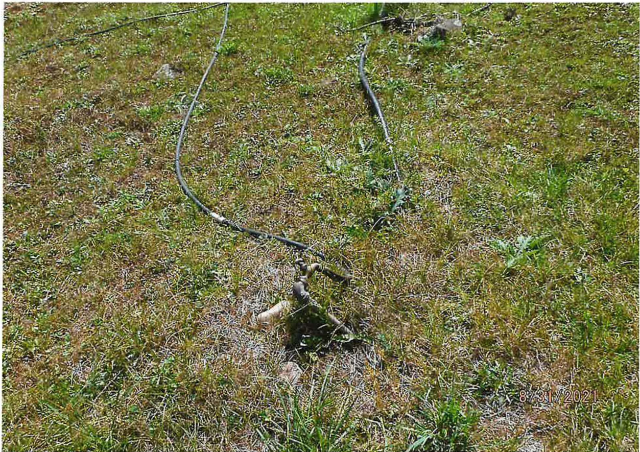
IRRIGATION POU – RISER PIPES TO HOSE BIB & SPRINKLER ATTACHMENTS
