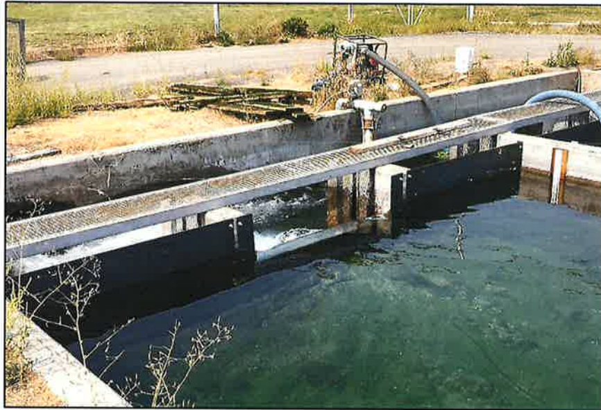
Figure 5. Left CTR raceway with weir plates and staff gauge.
