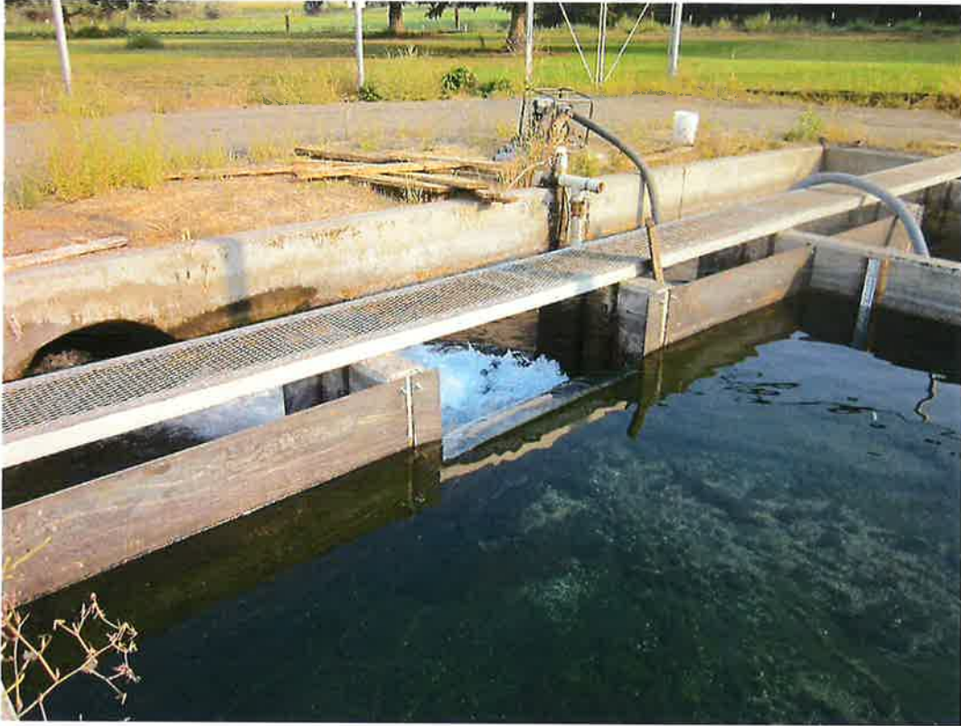
Figure 7: The 4.5' contracted rectangular weirs
