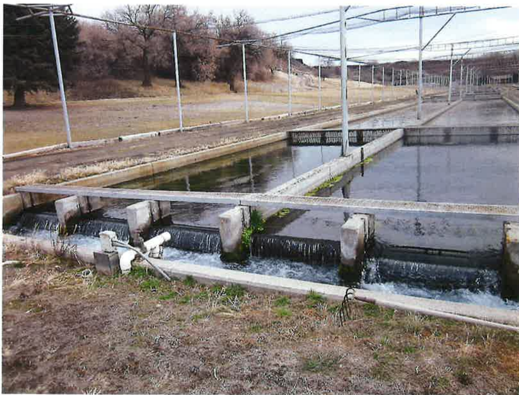
Figure 6: Lower Raceways prior to weir installation
