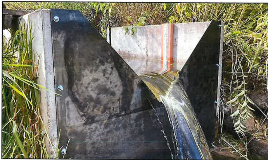
Figure 2. Upstream view of lodge pond dam V-notch weir.
