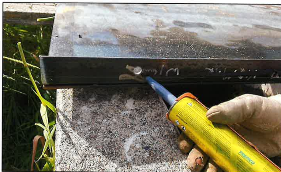
Figure 3. Application of waterproof sealant.
