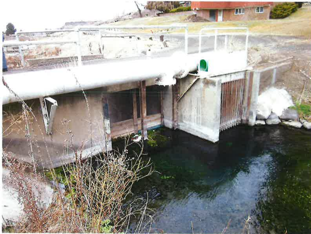
Figure 3: Bridge diversion (grated pipe intake) and check dam.
