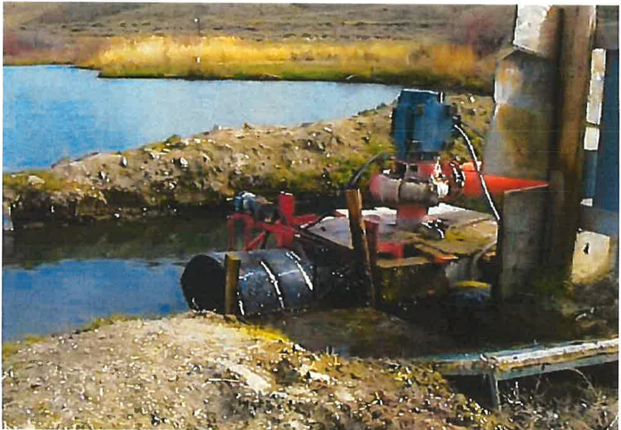
Settling pond (in background) and re-lift pump to canal (Photo from 5/9/2000 Tim Luke memo)
