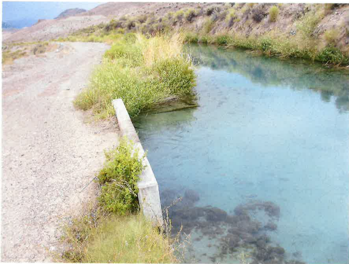
Intake from canal to fish facility
