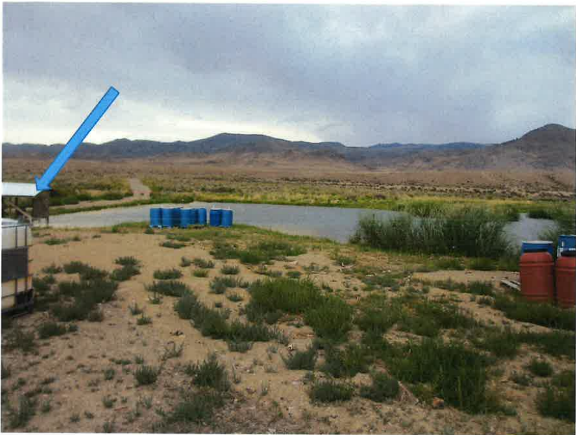
Settling pond – Pump at arrow
