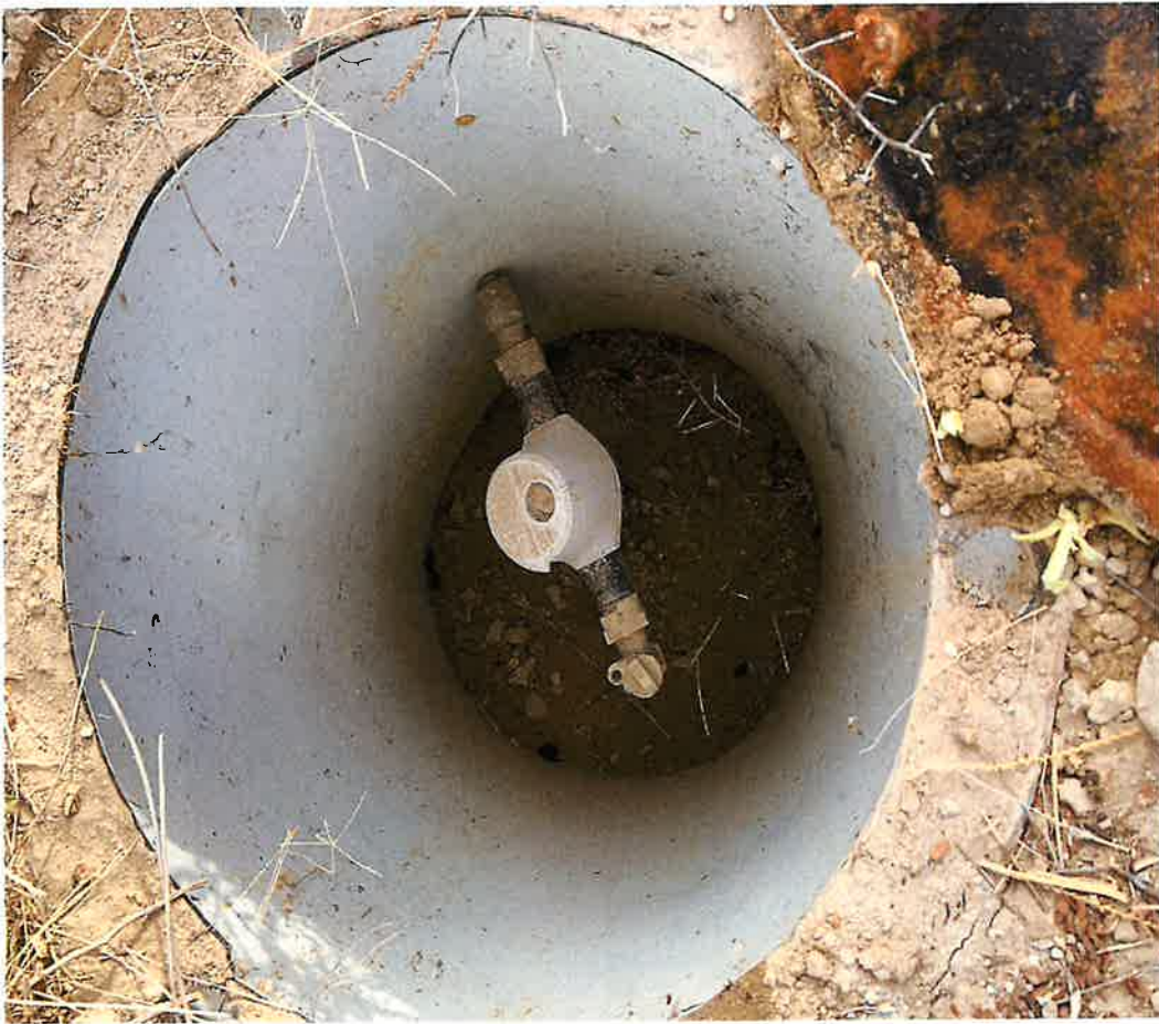
Fig. 14 – View of a “stub-in” for a lot in the West River Subdivision. All houses that are not already built or currently being built have been stubbed in.
