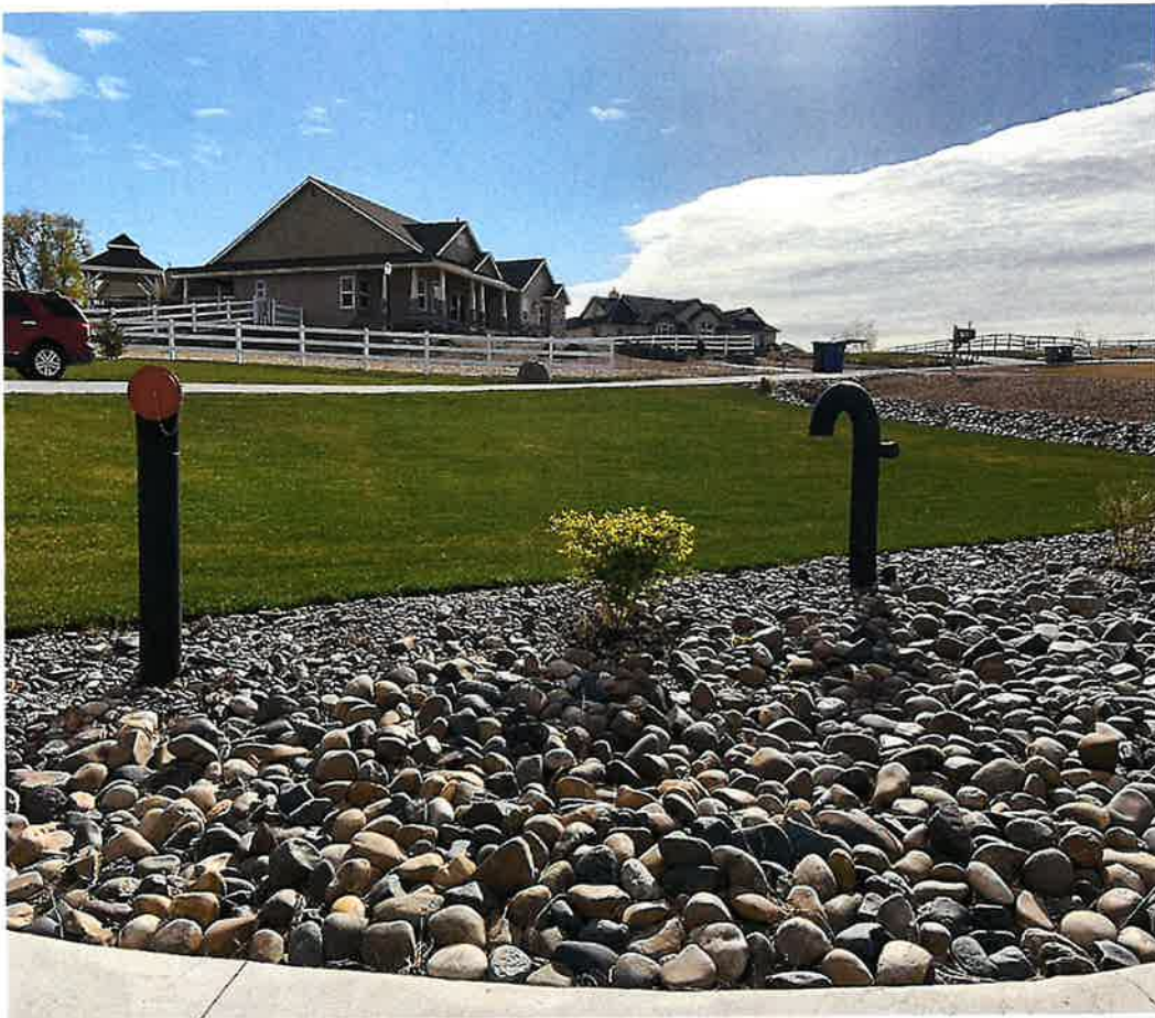
Fig. 16 – Access pipe for the fire protection tank buried on Lot 12, Block 2.
