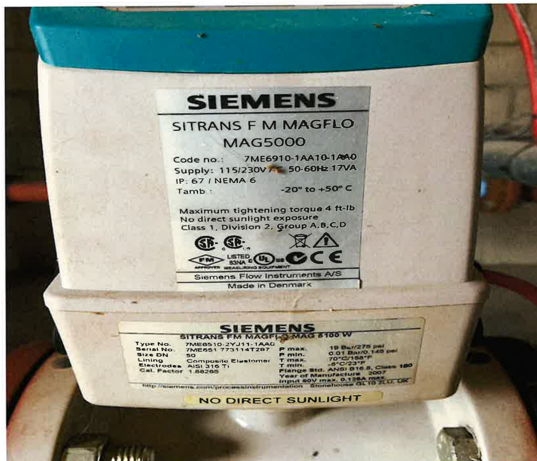
Fig. 6 – Specifications for Siemens inline device:
