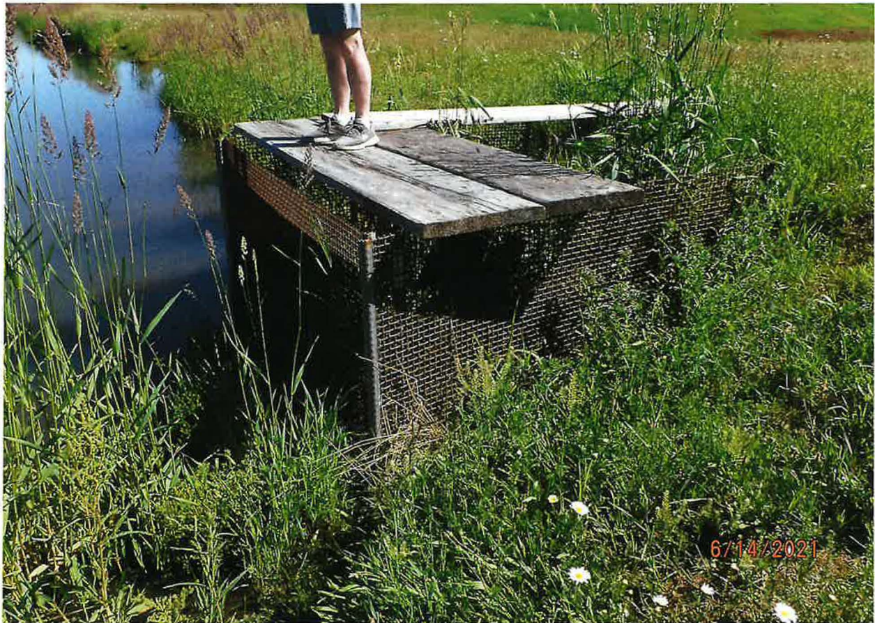
PRIMARY OVERFLOW DEVICE – CORRUGATED SCREENED PIPE
