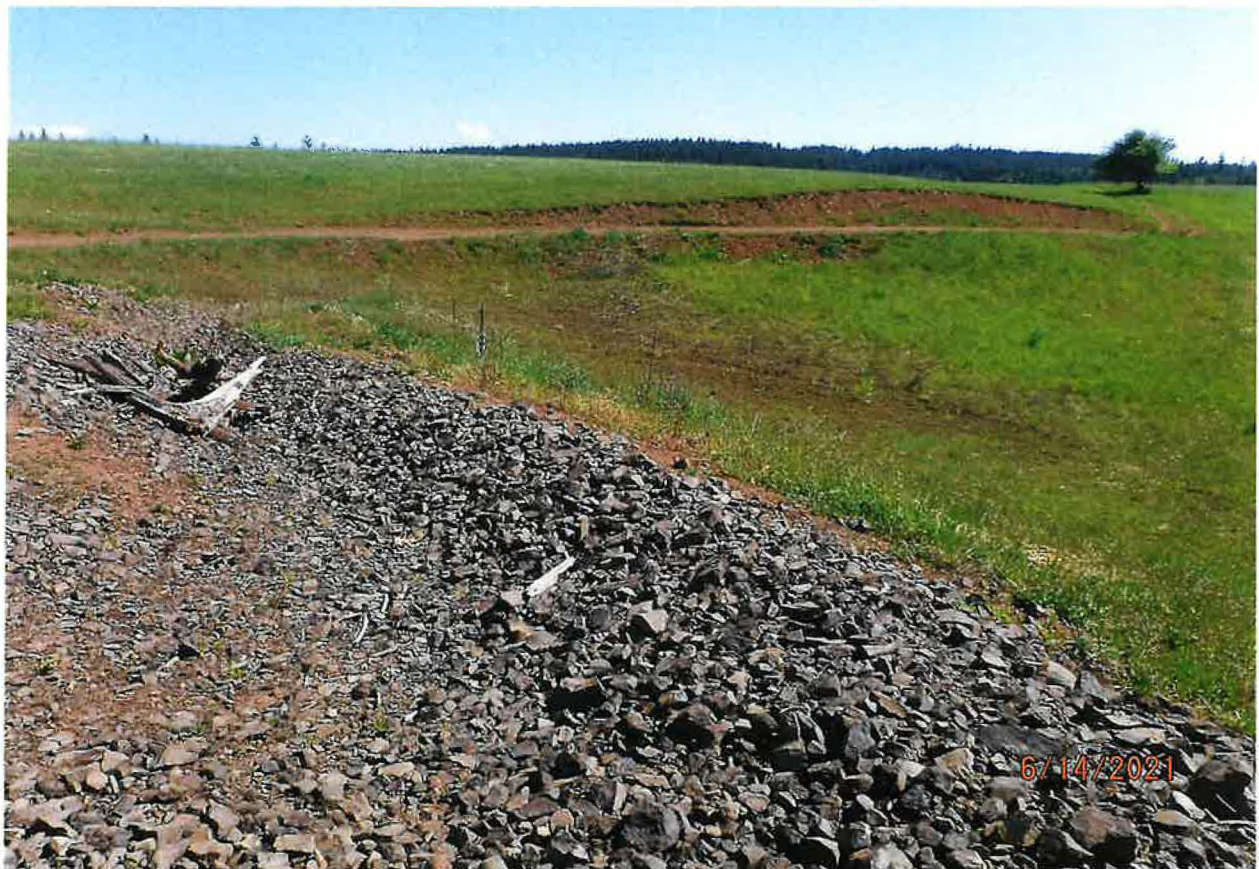
VIEW LOOKING DOWNGRADE FROM POND DAM
