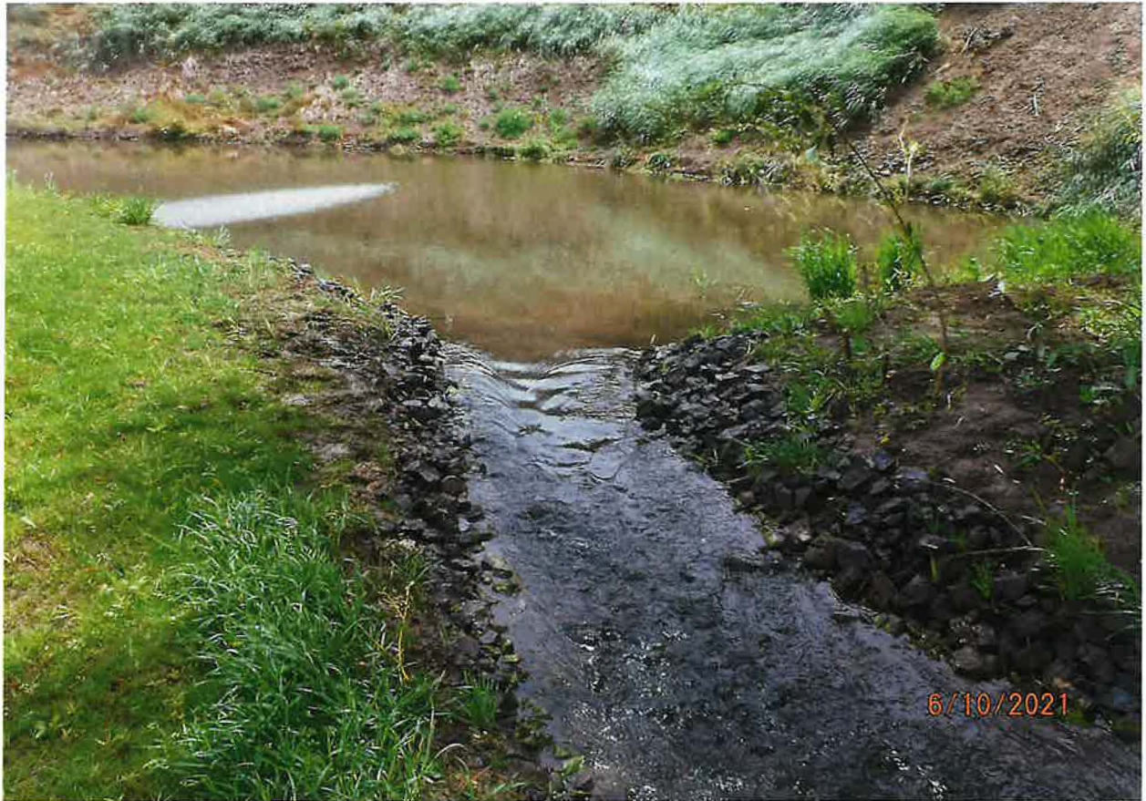
OUTFLOW FROM POND – ROCKED STREAM CHANNEL
