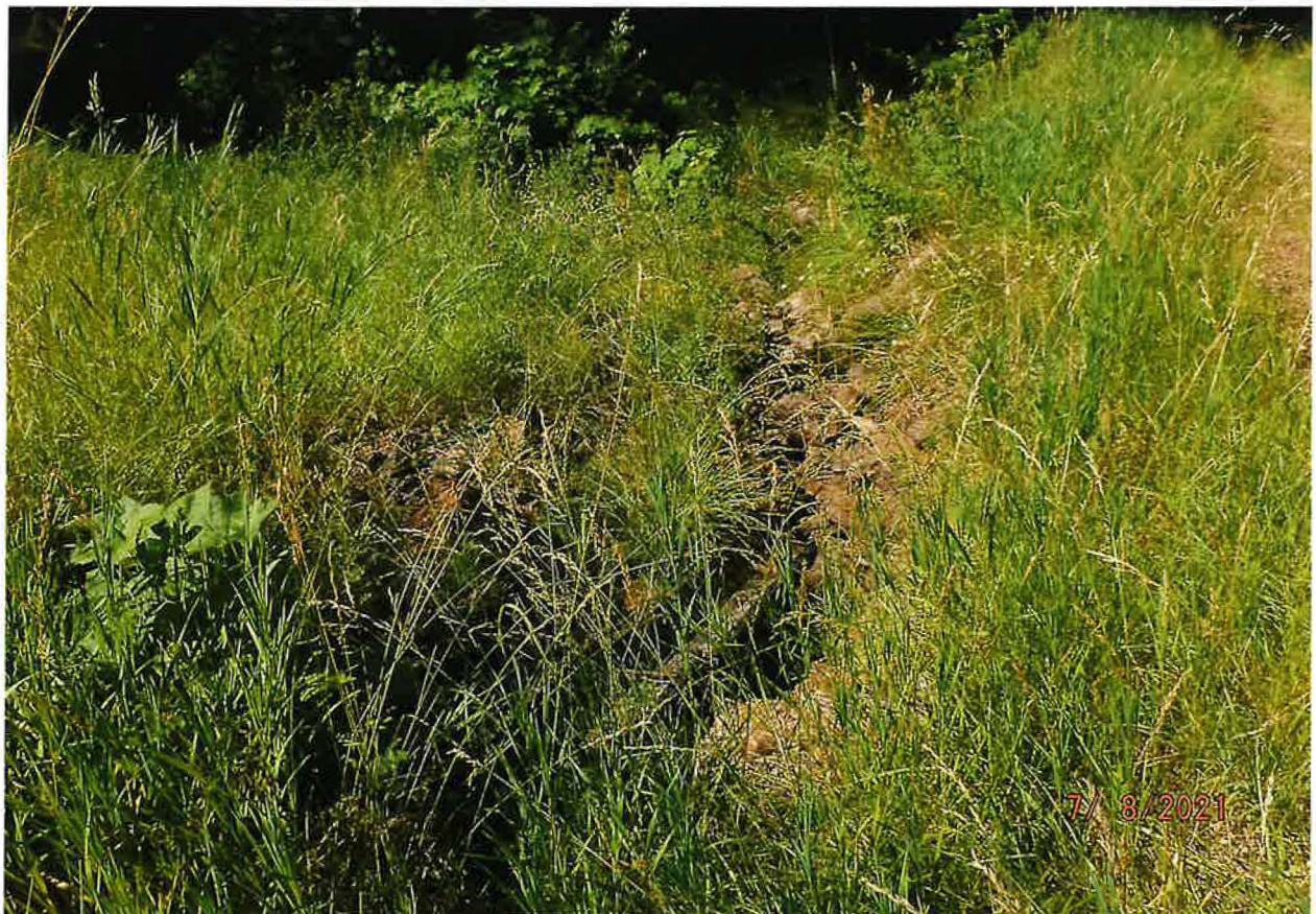
DOWNHILL SLOPE OF POND DAM – OVERFLOW PIPE DISCHARGES BACK TO STREAM CHANNEL
