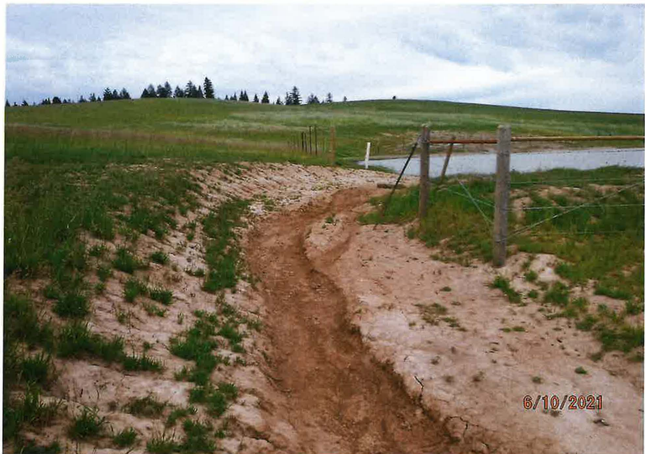
SECONDARY OVERFLOW CHANNEL (NW CORNER OF POND)
