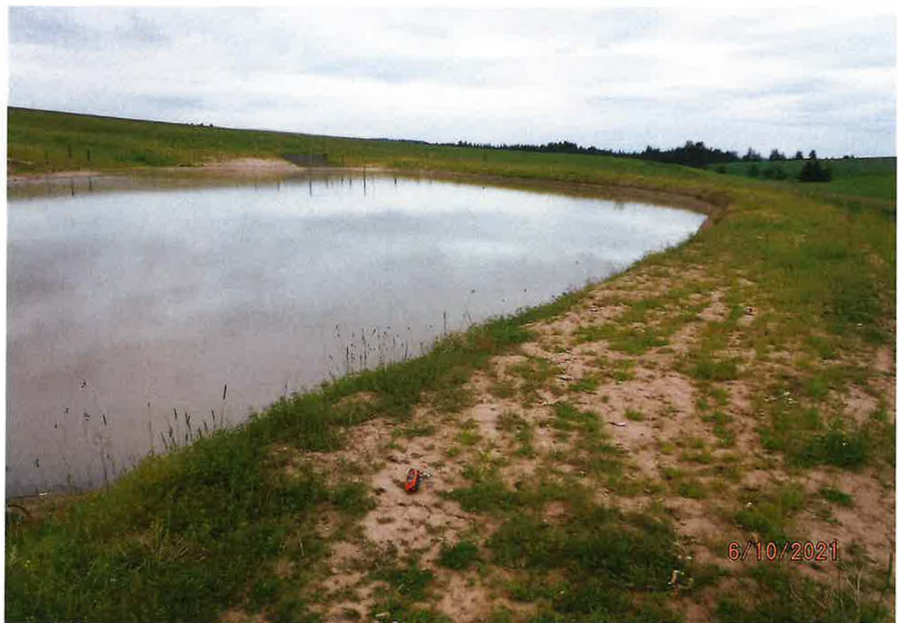
POD – POND EARTHEN DAM IMPOUNDS WATER FROM 2EA UNNMAED STREAMS
