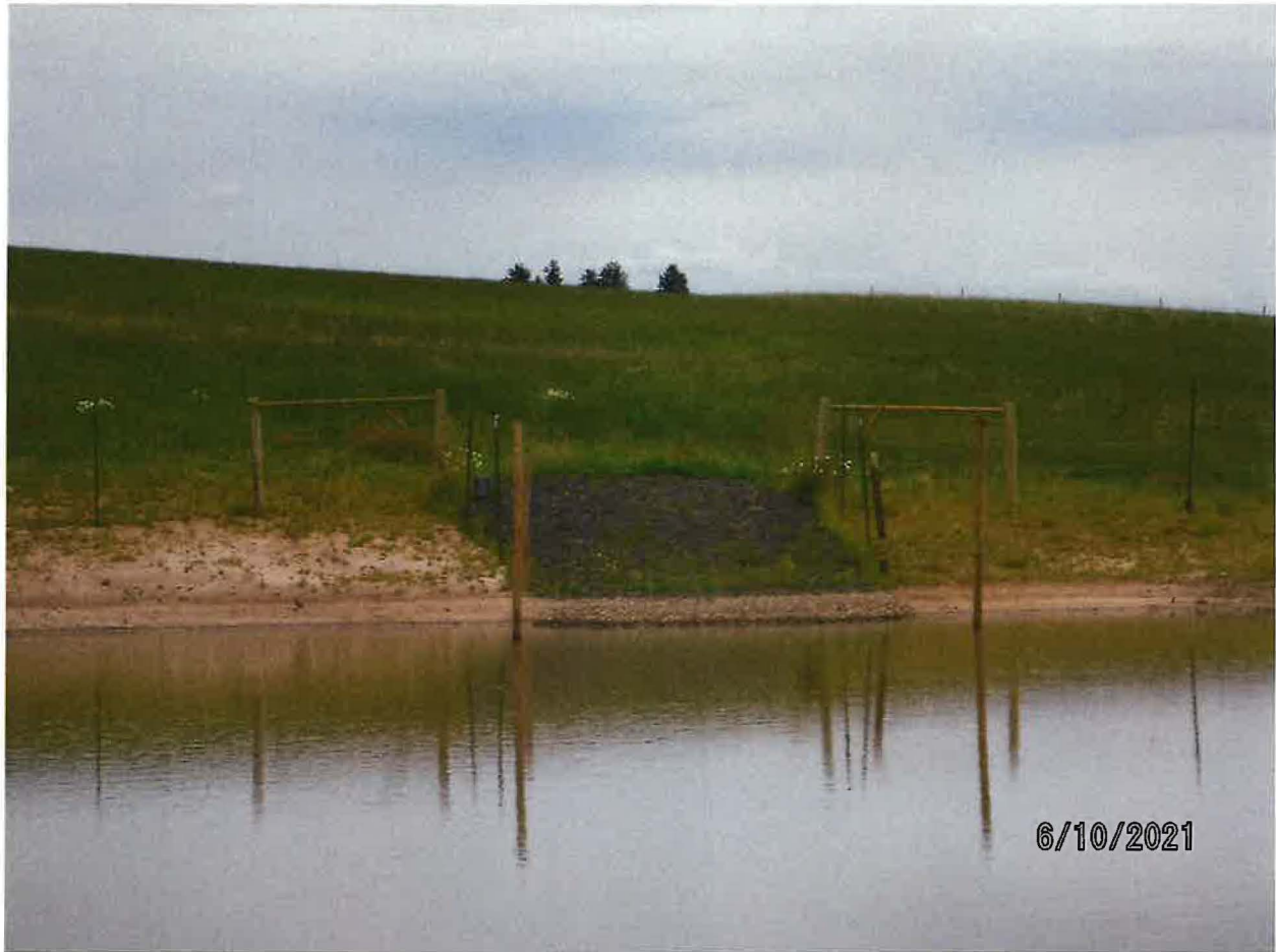
FENCED AND ROCKED STOCKWATER ACCESS TO POND – REST OF POND FENCED OFF TO PROTECT POND BANKS FROM STOCK
