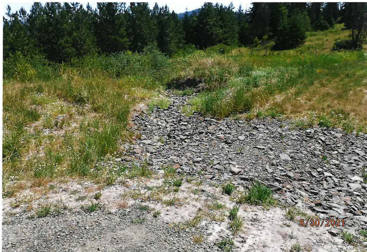
ROCKED OVERFLOW CHANNEL (DOWN STREAM SIDE OF DAM VIEW)
