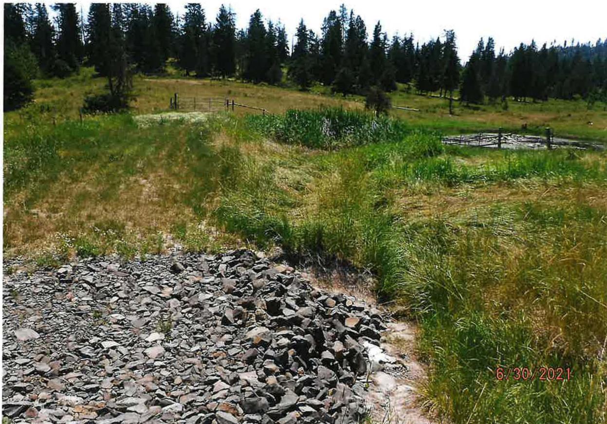
BASALT ROCKED OVERFLOW CHANNEL (POND SIDE OF DAM VIEW)
