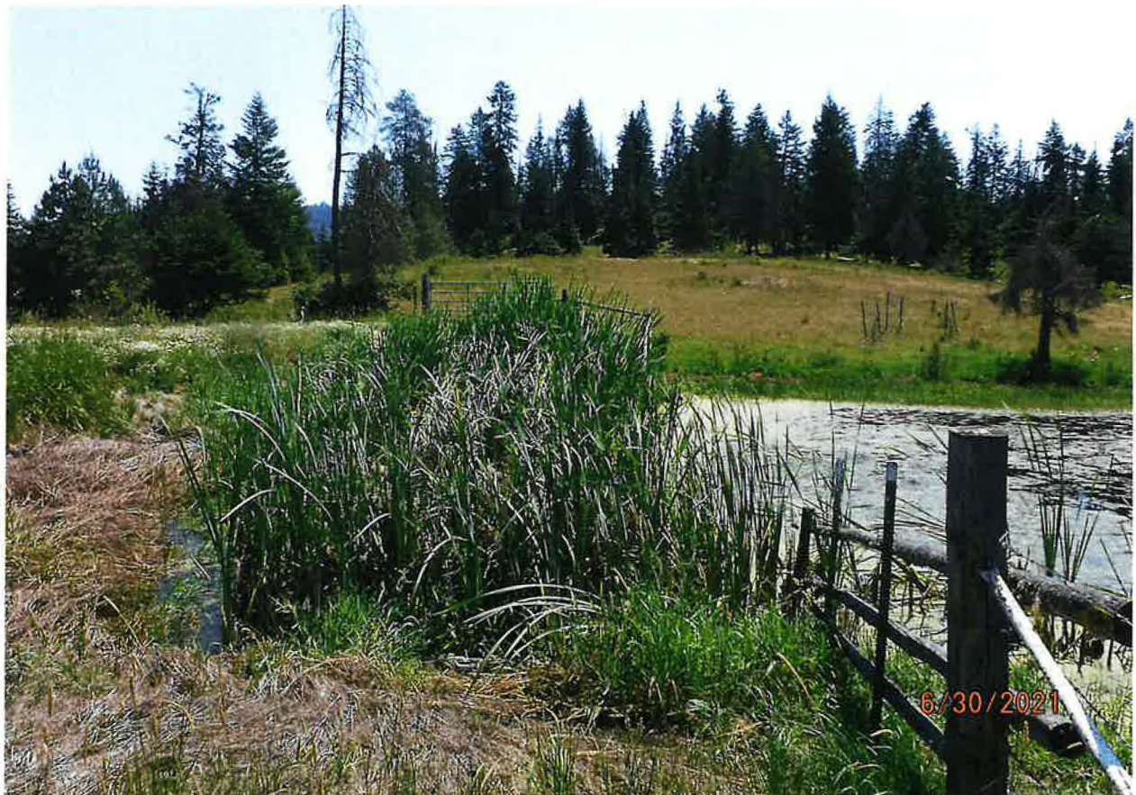
FENCE INSTALLED TO PREVENT STOCK FROM DETERIORATING POND DAM/ROADWAY
