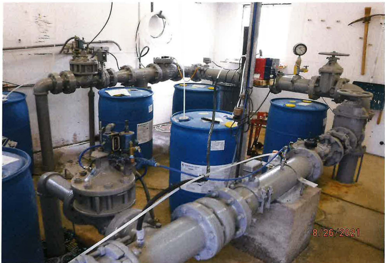
SYSTEM DIVERTING WORKS – COMMON SERVICE LINE TO SYSTEM FED BY 2 WELLS (R/H SIDE OF FRAME)
