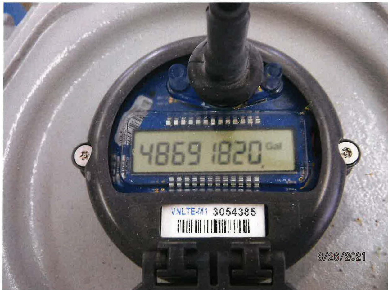
INSTANT REPORTING FLOWMETERS INSTALLED ON EACH MAIN INTAKE PIPE FROM WELL(S)
