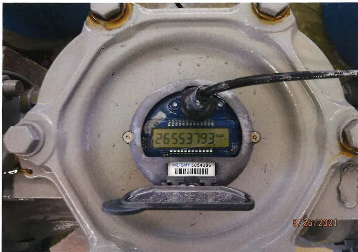
INSTANT REPORTING FLOWMETERS INSTALLED ON EACH MAIN INTAKE PIPE FROM WELL(S)
