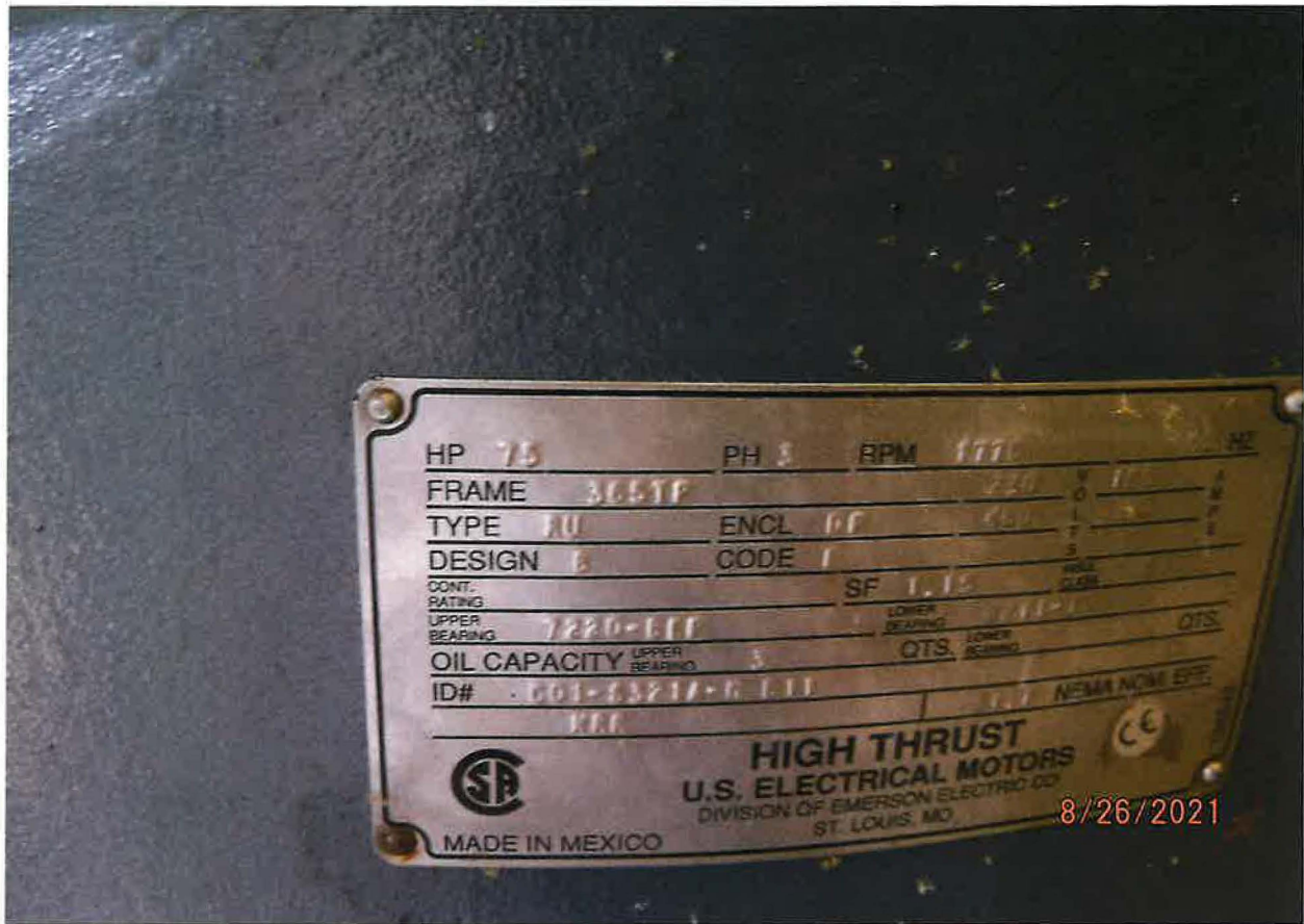
WELL #1 – 75 HP PUMP MOTOR INSTALLED
