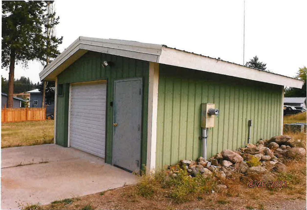
PUMP STATION, WELL #1 LOCATED INSIDE
