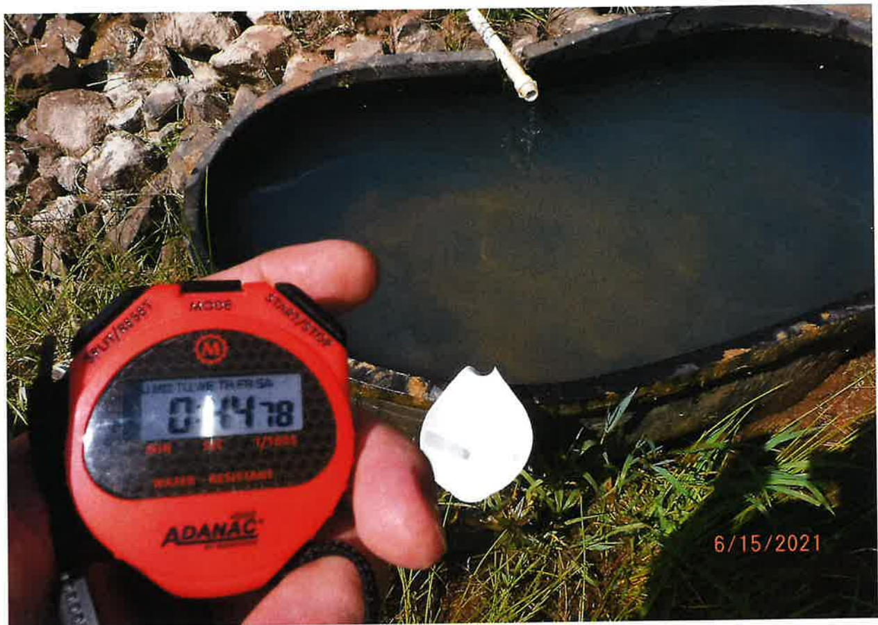
4 CUP MEASURING DEVICE USED TO CAPTURE FLOW MEASUREMENT FROM TANK OVERFLOW PIPE
