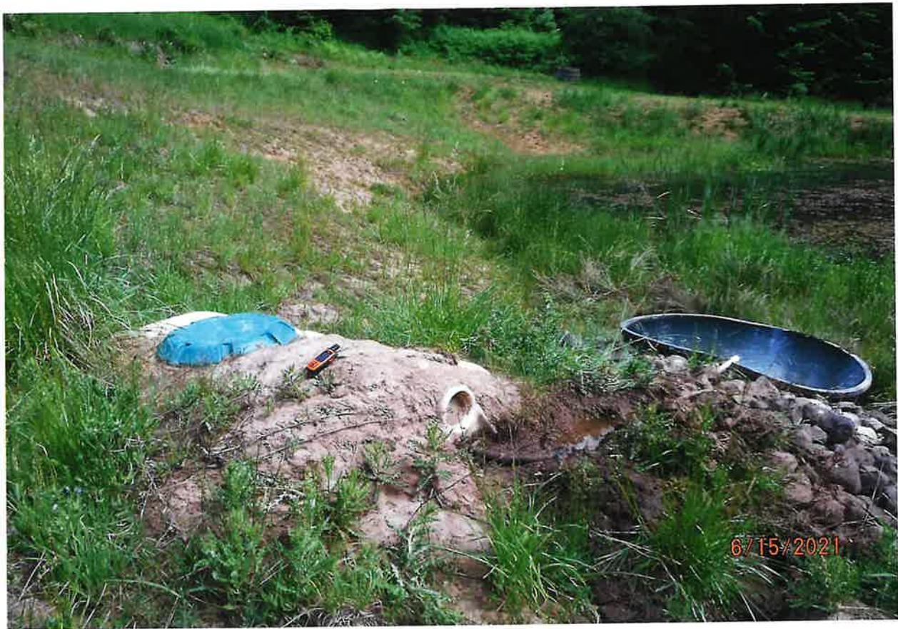
600 GALLON STORAGE TANK CAPTURES SPRING FLOW & ROUTES TO TROUGH
