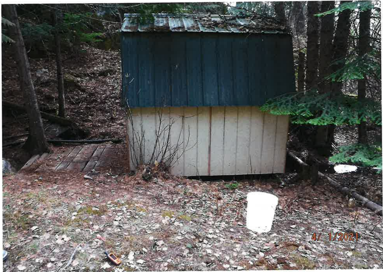
POWER HOUSE CONTAINING HARRIS HYDRO UNIT
