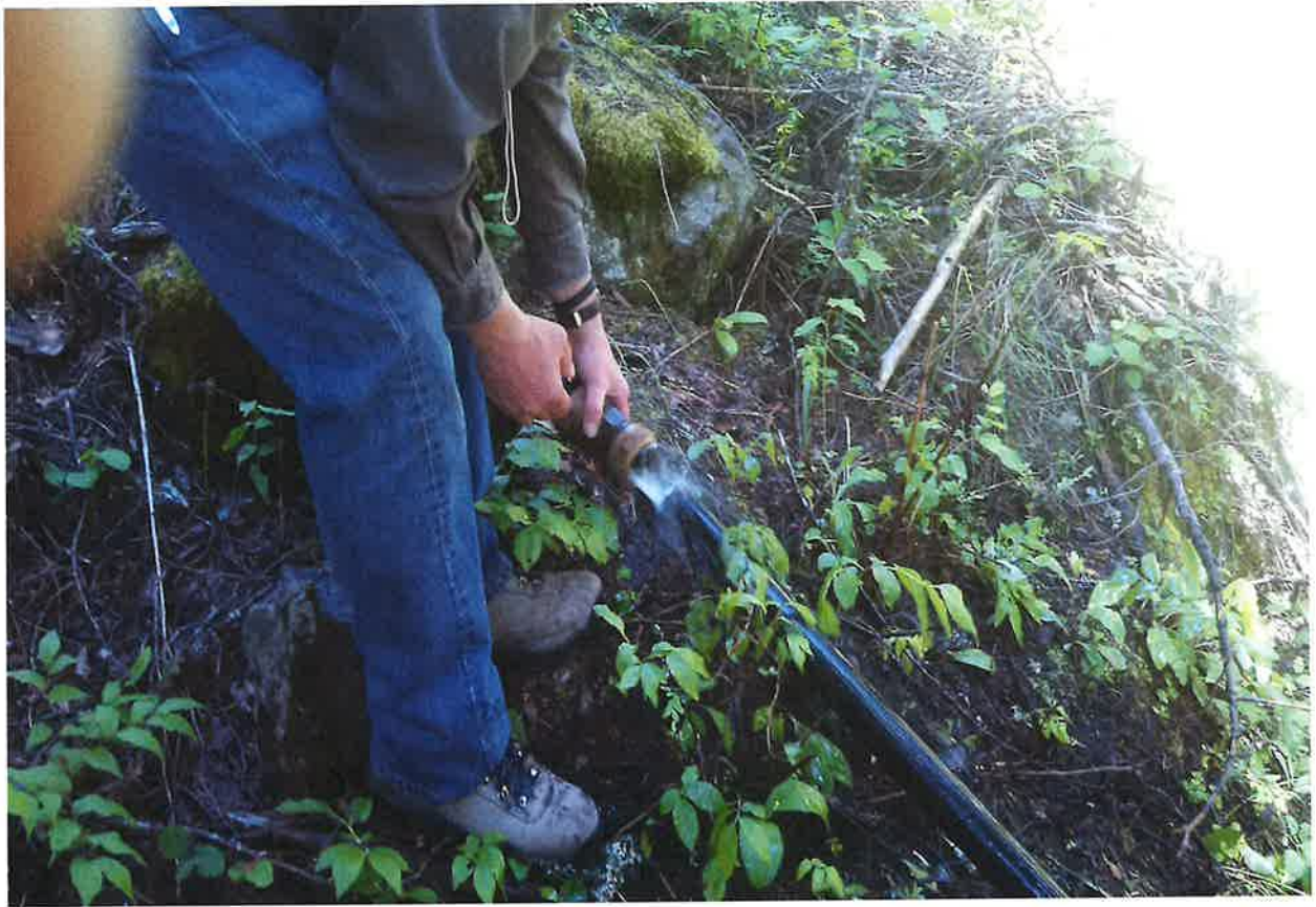
2 INCH POLY PIPE ROUTED FROM POD-TO-POWER HOUSE
