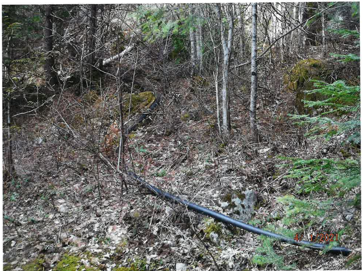
2 INCH POLY PIPE ROUTED FROM POD-TO-POWER HOUSE
