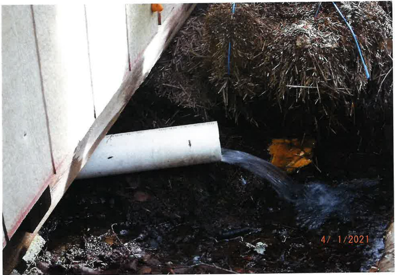
OVERFLOW DISCHARGE FROM HARRIS HYDRO UNIT
