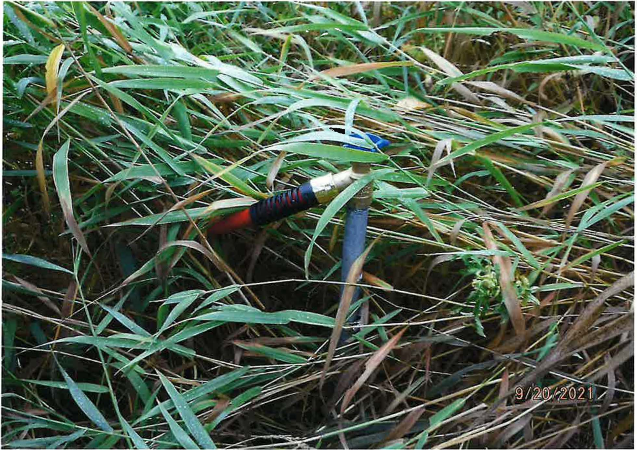
END OF \frac{3}{4} INCH POLY PIPE RUN – TO – \frac{1}{2} INCH RISER PIPE AND HOSE BIB ATTACHMENT
