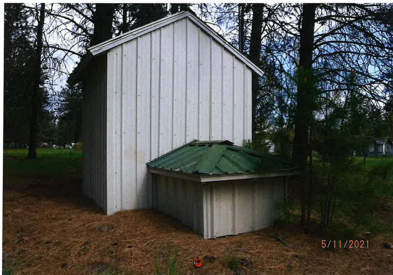
PUMP HOUSE & WELL (COVERED DOGHOUSE)
