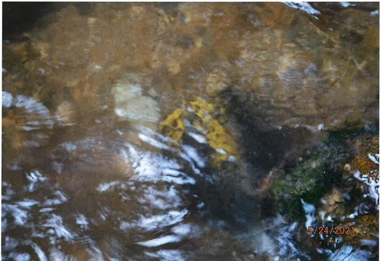
POD – SCREENED INTAKE PIPE IN CREEK
