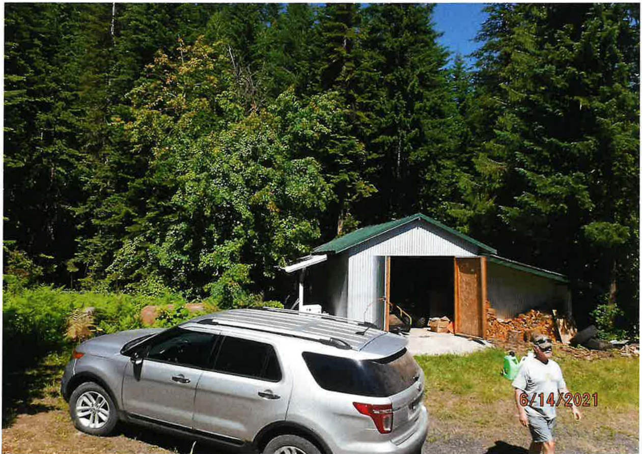
SMALL SHED – HOUSES STORAGE TANK CO-LOCATED WITH HOUSE FOR DOMESTIC WATER USE
