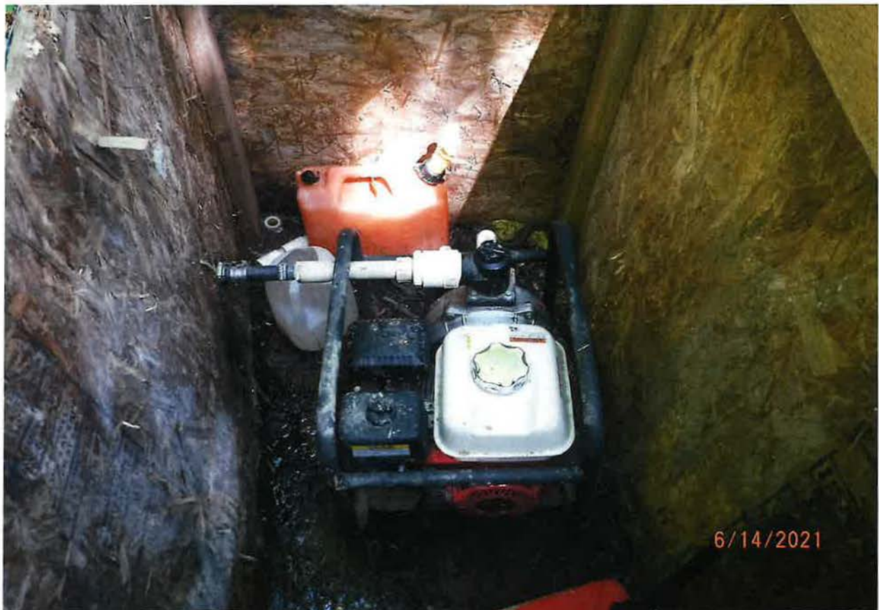
PUMP ENCLOSURE, HOUSES SMALL WATER TRANSFER PUMP
