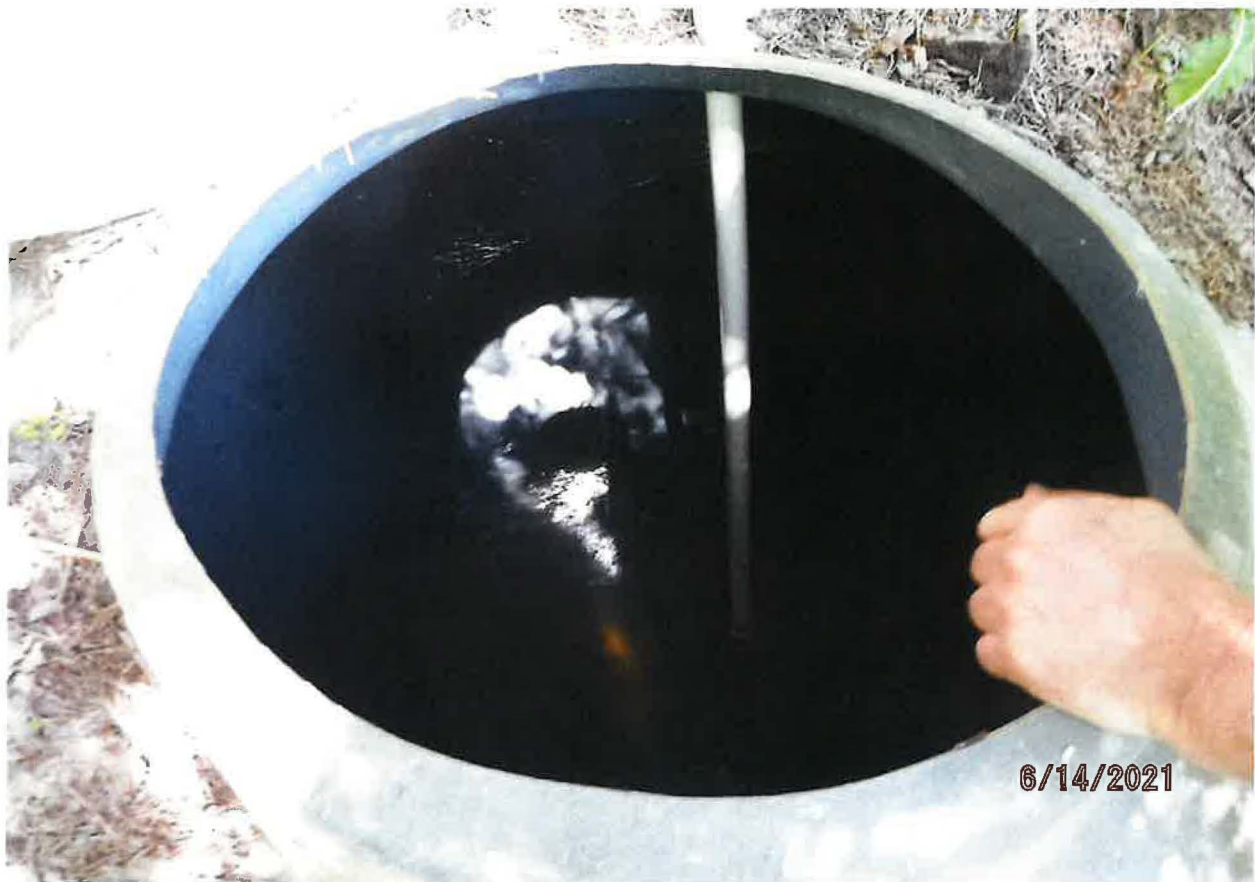
POD – SPRING SOURCE – STORAGE TANK CAPTURES WATER FROM A BURIED PERFORATED PIPE
