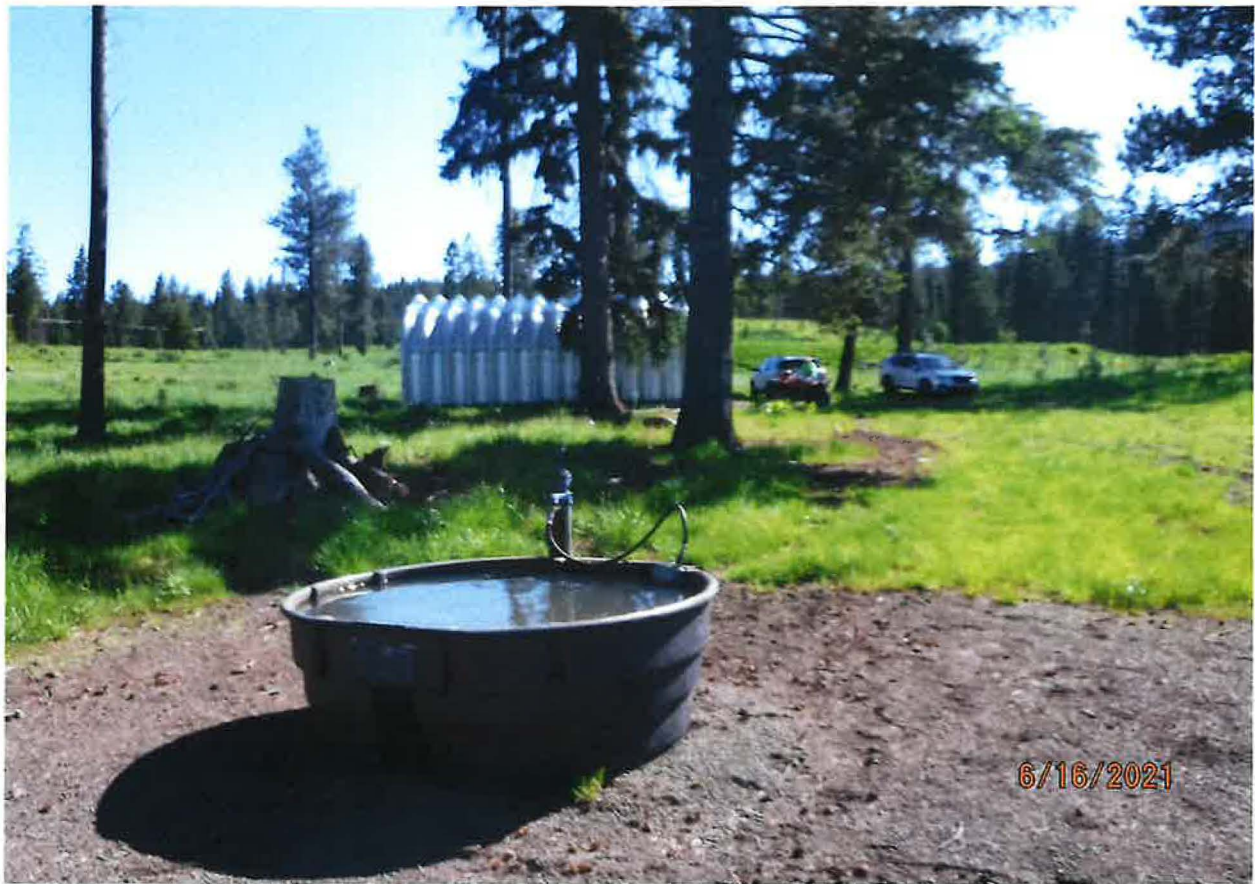
STOCKWATER FROM STORAGE USE – PIPE ROUTED FROM POND TO FROST FREE HYDRANT AND TANK
