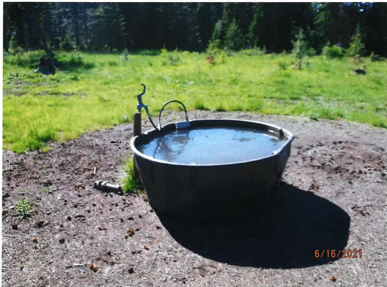
STOCKWATER FROM STORAGE USE – PIPE ROUTED FROM POND TO FROST FREE HYDRANT AND TANK
