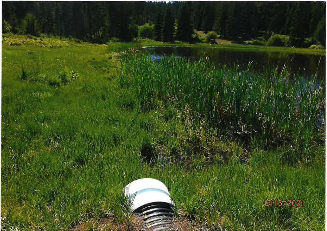
OVERFLOW DISCHARGE PIPE FROM POND
