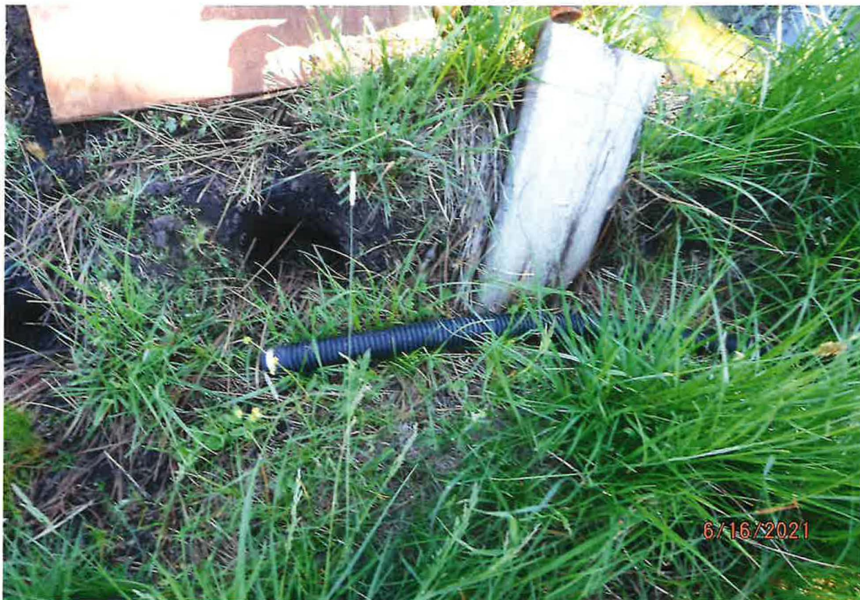
CONNECTOR TUBE USED TO FILL TRAILER TRANSPORTED WATER TANK
