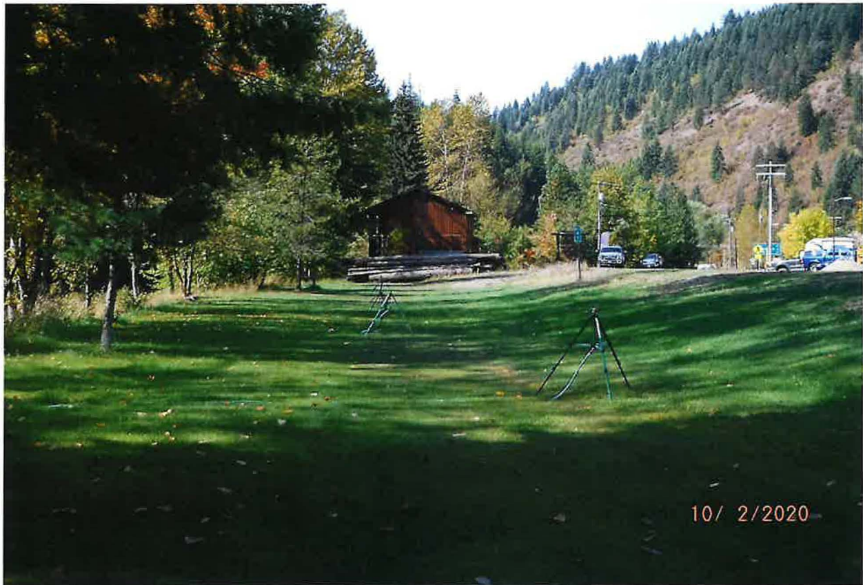
FIRE PROTECTION & IRRIGATION POU – LOOKING WEST FROM TEE IN WATER LINE
