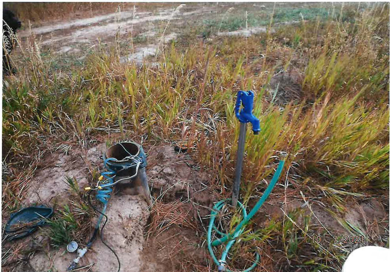
POD – GROUNDWATER WELL (WIRING REPAIR IN PROCESS AT TIME OF EXAM)
