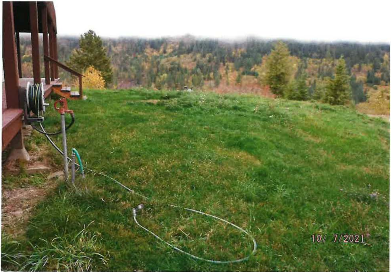
IRRIGATION POU – STUB PIPE WITH HOSE ROUTES TO IRRIGATION JUNCTIONS' DOWNHILL
