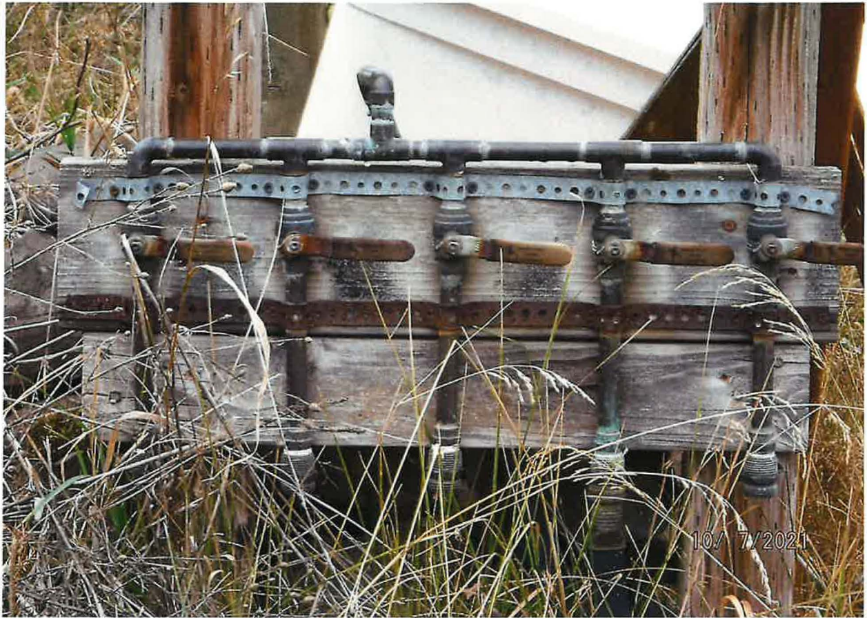
IRRIGATION POU – WATER ZONE SPLITTER PANEL
