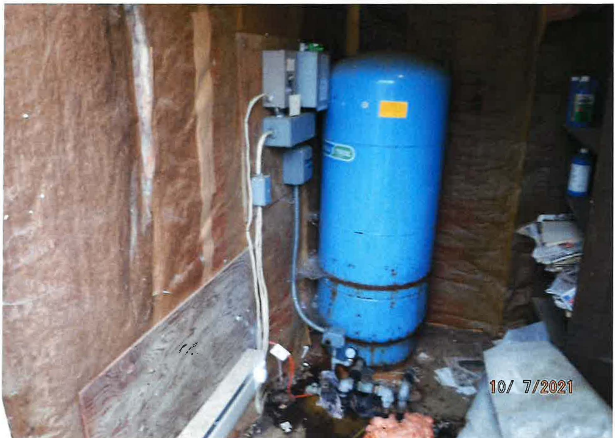
WATER SYSTEM DIVERTING WORKS
