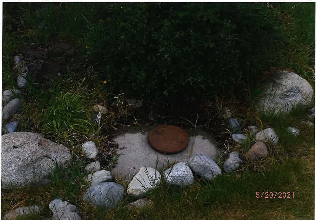
Capped Well #2, no pump installed at time of field exam
