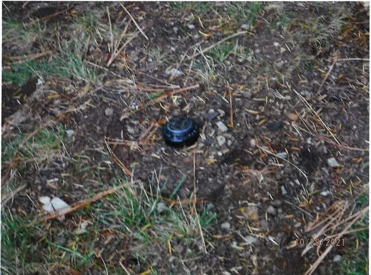
IRRIGATION POU – LAWN SPACE USES PRESSURIZED RAINBIRD SPRINKLER SYSTEM
