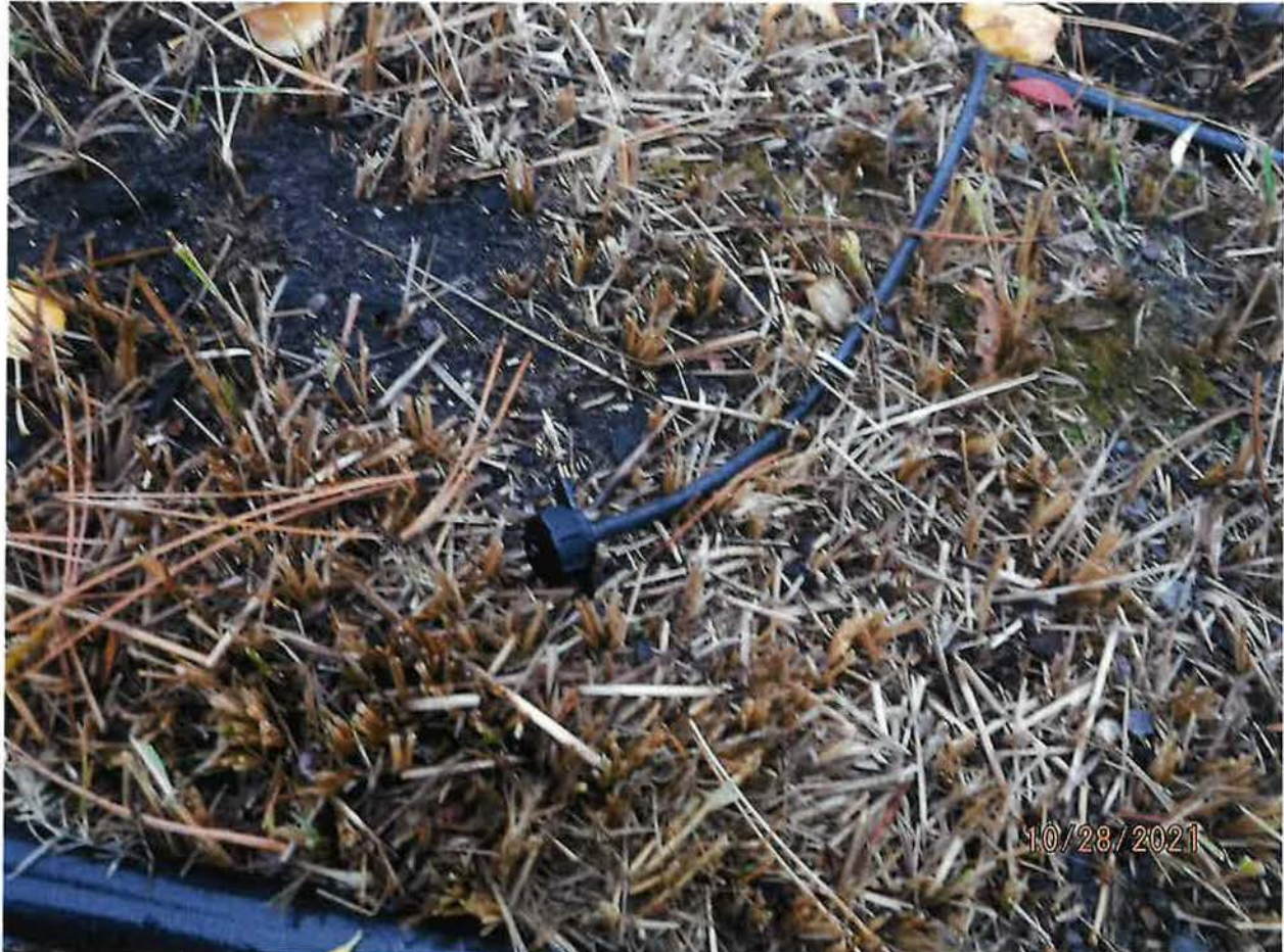
IRRIGATION POU – LANDSCAPE AND TREE WATERING BY PRESSURIZED SYSTEM, MICRO EMITTERS
