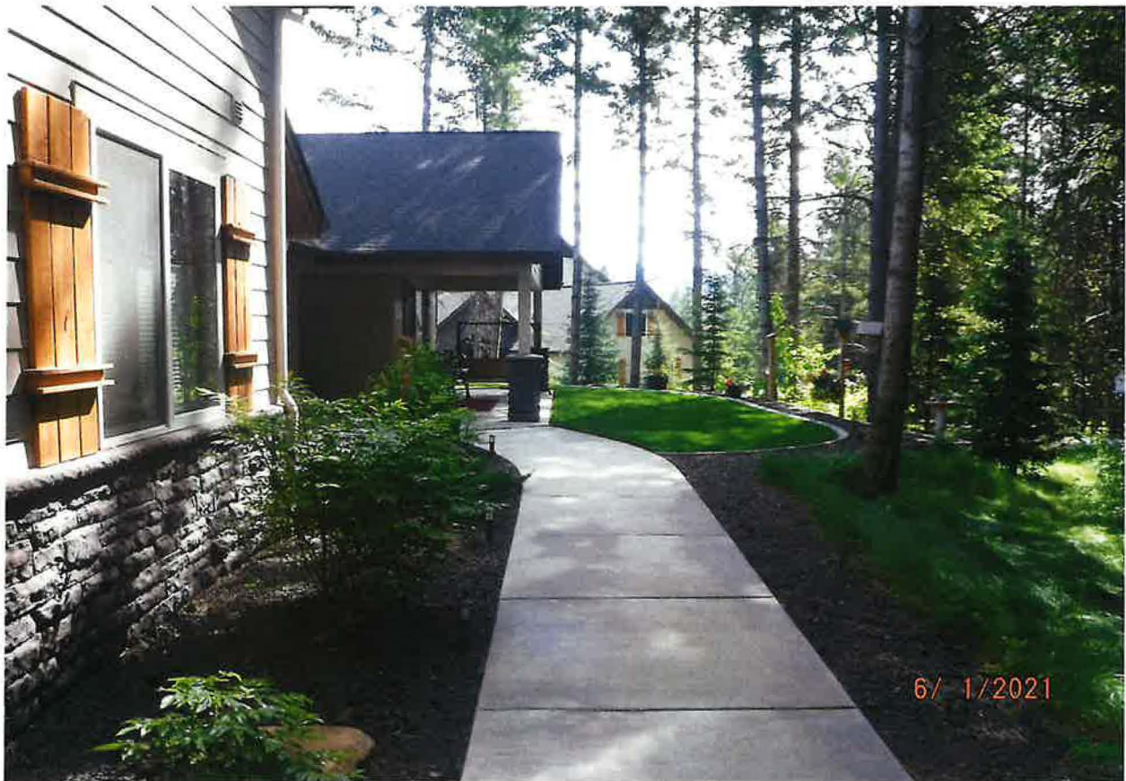
IRRIGATION POU – PRESSURIZED SPRINKLER SYSTEM
