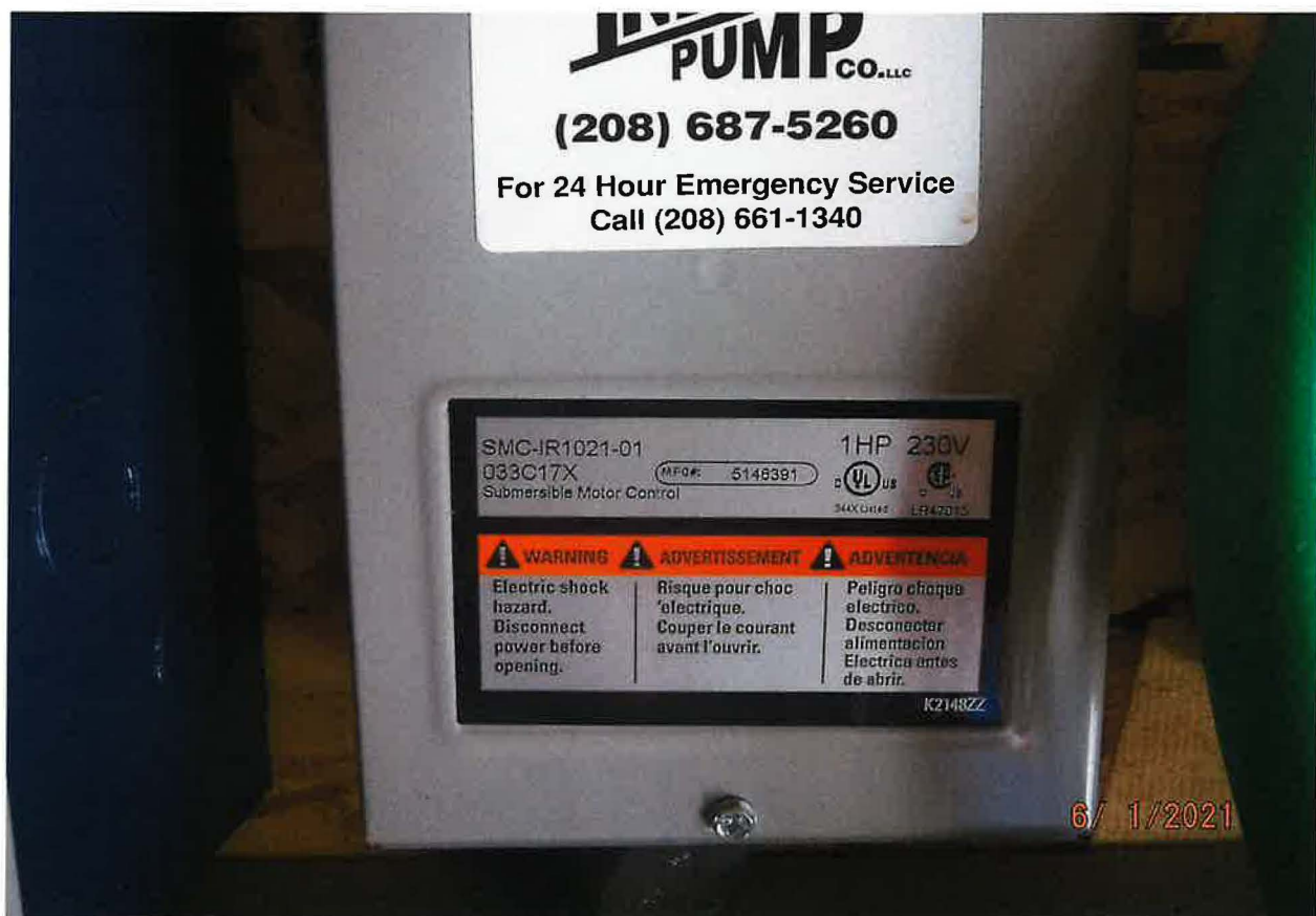
WELL PUMP 5 HP 3 PHASE (NO DATA PLATE); TRANSFER PUMP FROM STORAGE TANK(S)-1 HP
