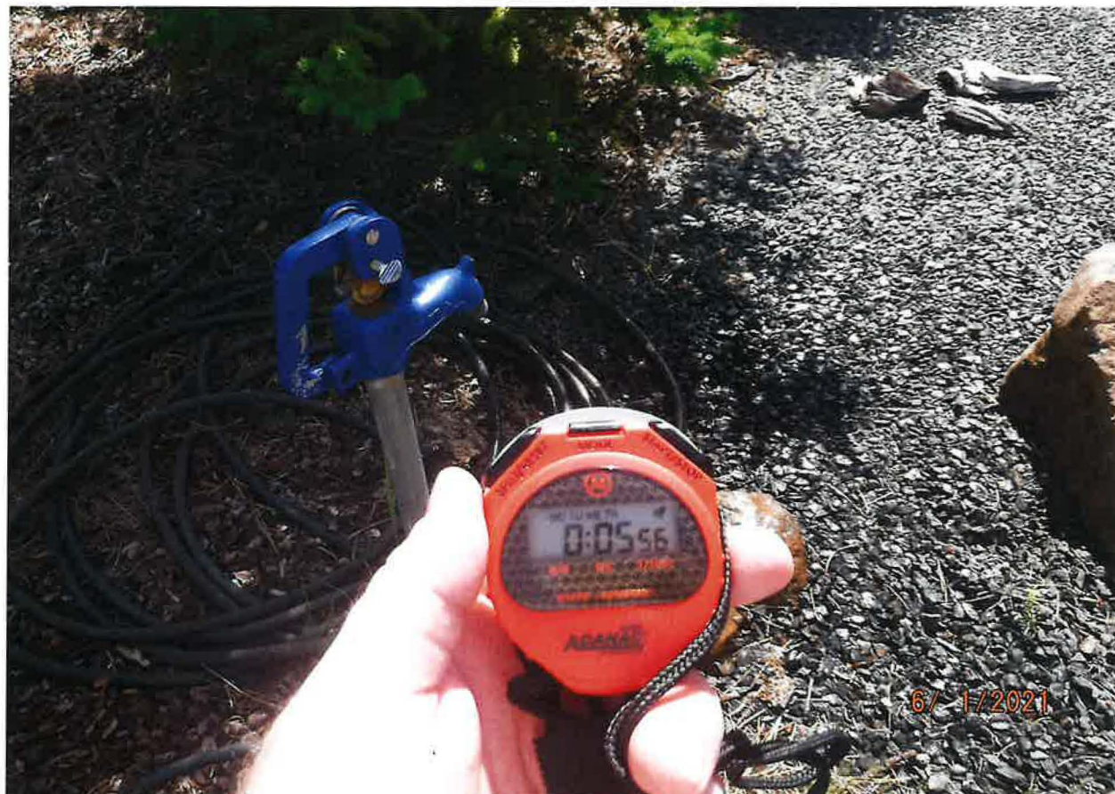
FROST FREE HYDRANT CO-LOCATED WITH WELL
