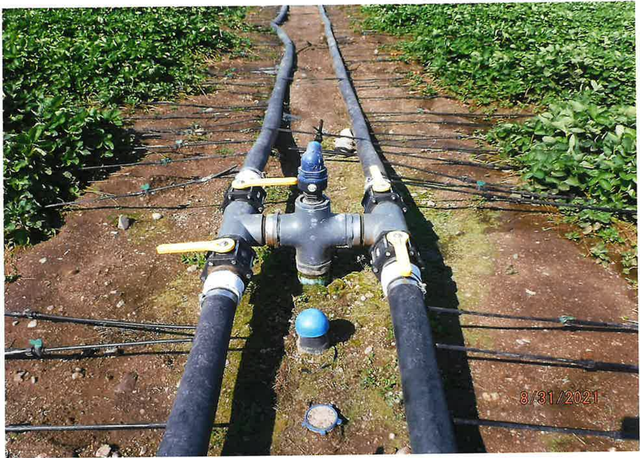
IRRIGATION RISER PIPE TO SOAKER HOSE SYSTEM AT INTERVAL ALONG NORTHERN EXTENT OF POU
