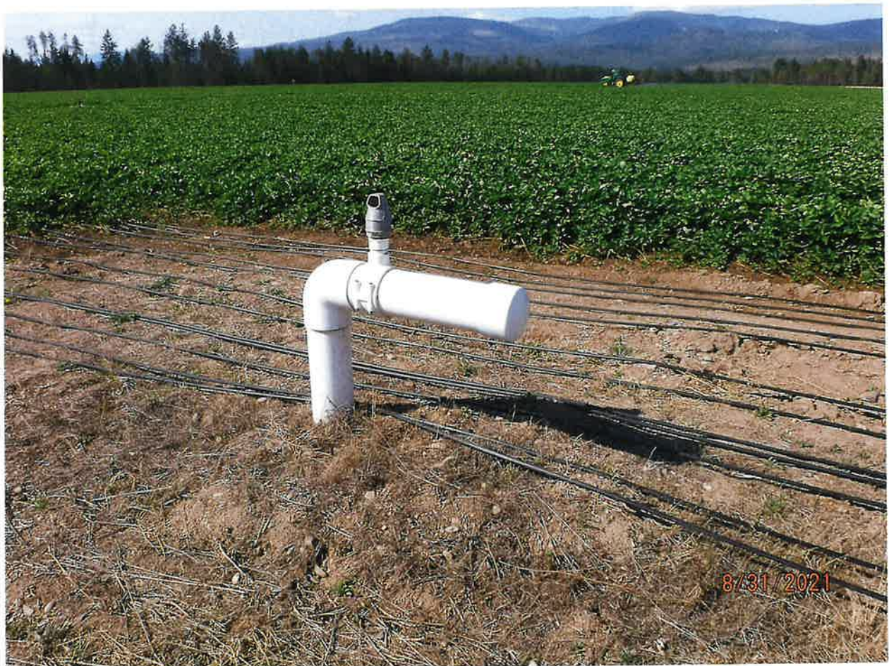
BURIED IRRIGATION MAIN LINE WITH RISERS
