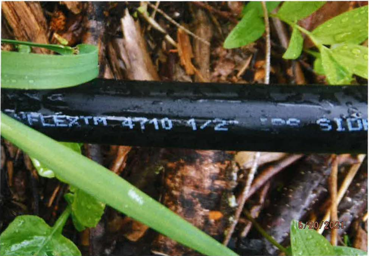
½ INCH DELIVERY PIPE FROM RAM PUMP TO STORAGE TANKS
