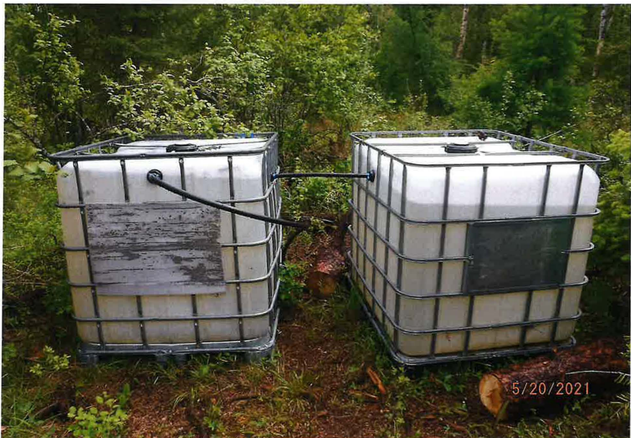
DISCHARGE LINE FROM L/H TANK RETURNS OVERFLOW WATER BACK TO CREEK
