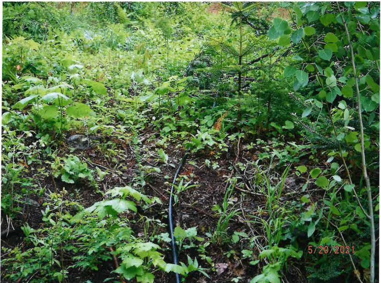
½ INCH DELIVERY PIPE FROM RAM PUMP TO STORAGE TANKS
