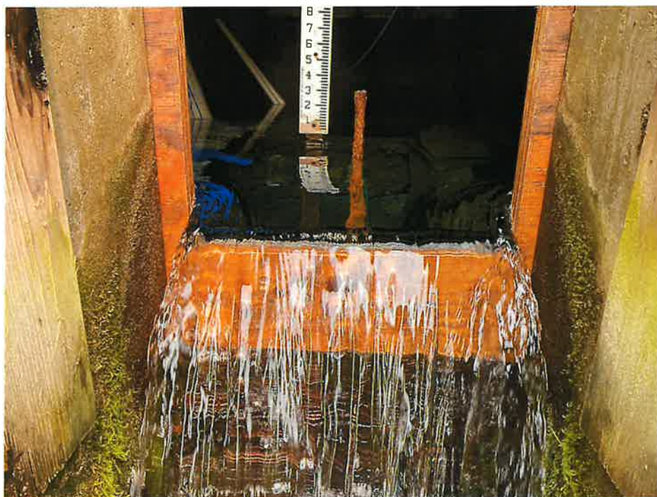
Figure 8. 18-inch rectangular weir temporarily installed in check gate of IDFG Spring Box. Blue plastic sheeting was used to limit leakage through and around check boards below weir. The pressure transducer was clamped to a steel rod welded to a metal plate set behind the staff gauge (not visible in photograph).
