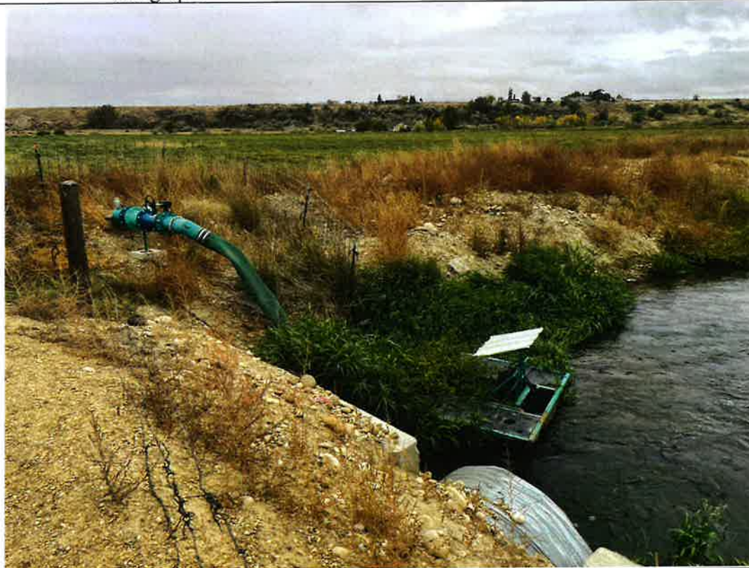
Floating Diversion on North Drain.
