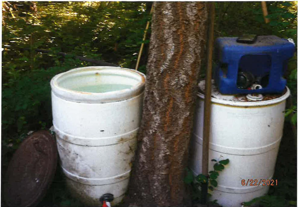
AT POD – 2EA 50 GAL DRUMS USED TO CAPTURE SPRING WATER
