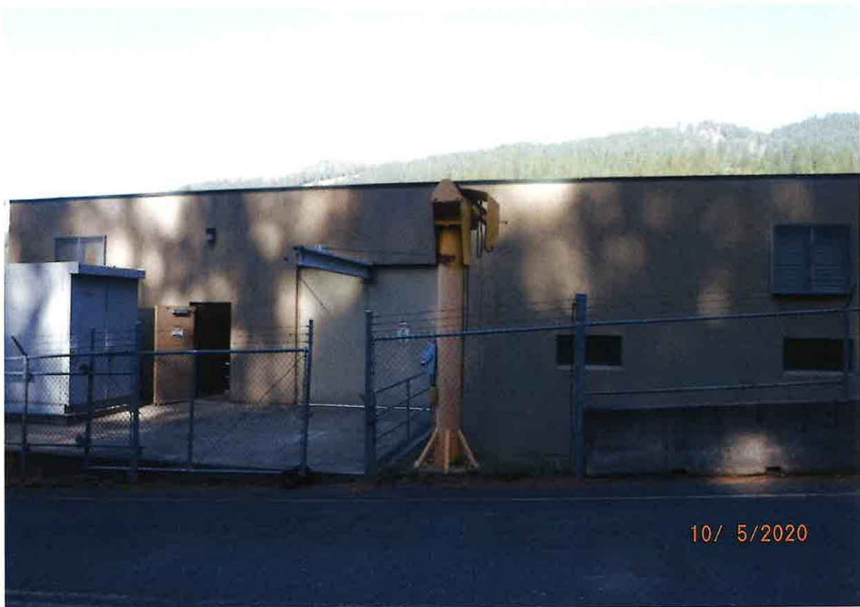
HYDRO POWER STATION
