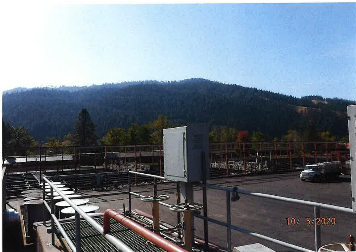
FISH PROPAGATION POU – WATER CONTROL TOWER
