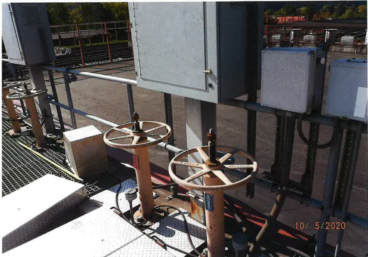
PRIMARY AND SECONDARY CONTROL VALVES (EXAMPLE)
