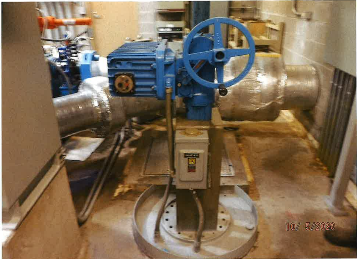
SECONDARY PAN SLEEVE VALVE FOR MANUAL OPERATION
