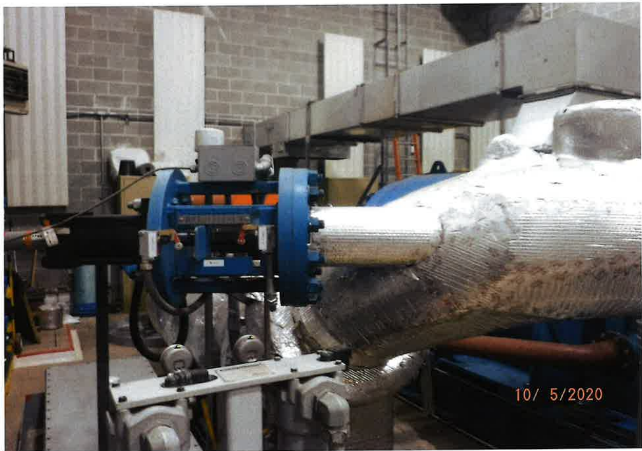
GATE VALVE INSTALLED ON PRIMARY PIPE
