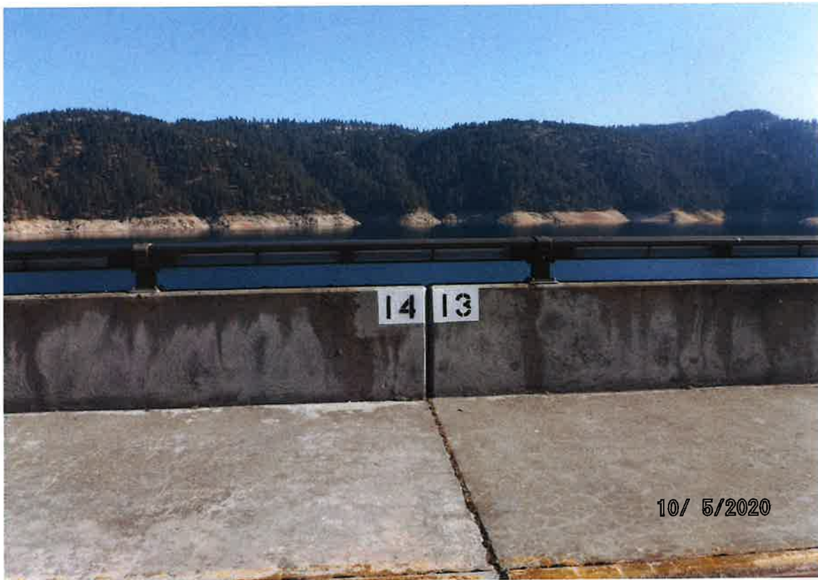
POD – SECONDARY SUBMERGED PIPE FIXED ALONG DAM SURFACE; GPS POINT TAKEN ON TOP OF DAM
