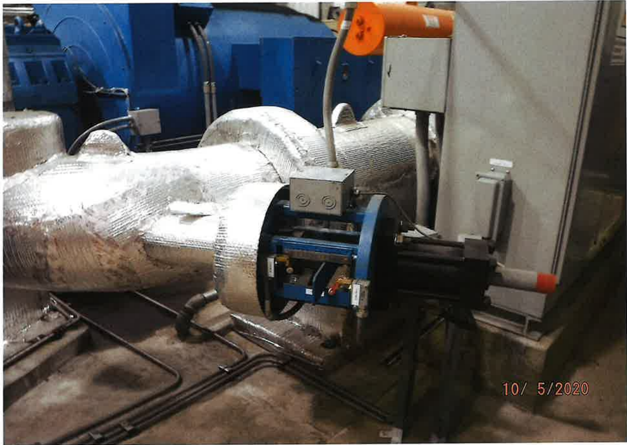
GATE VALVE INSTALLED ON SECONDARY PIPE
