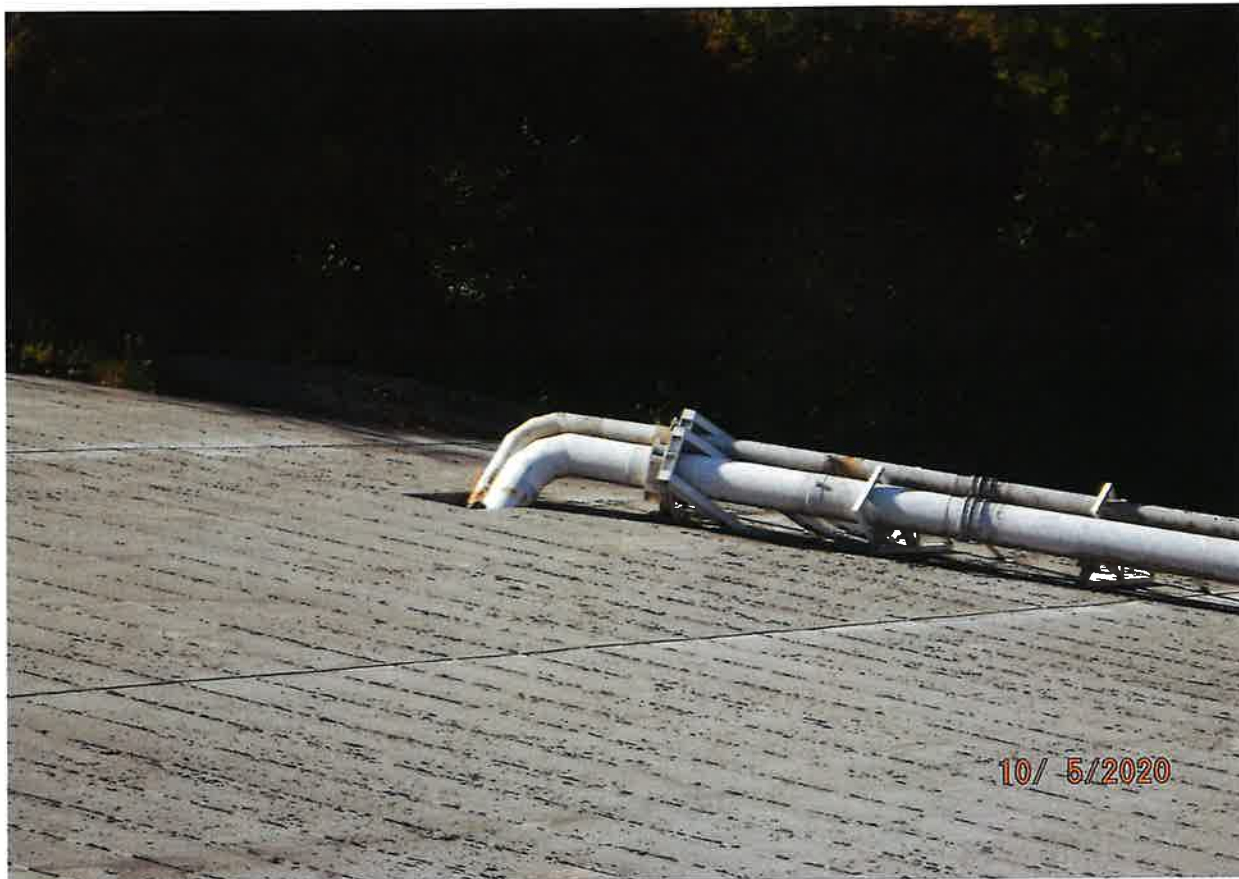
PRIMARY & SECONDARY PIPING EXITING DAM ON DOWNRIVER SIDE
