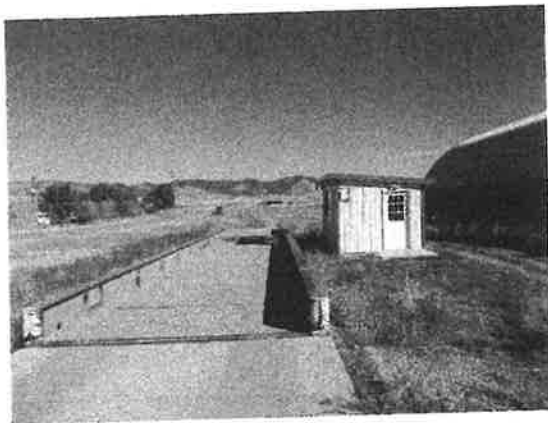
Truck scale adjacent to cellars
