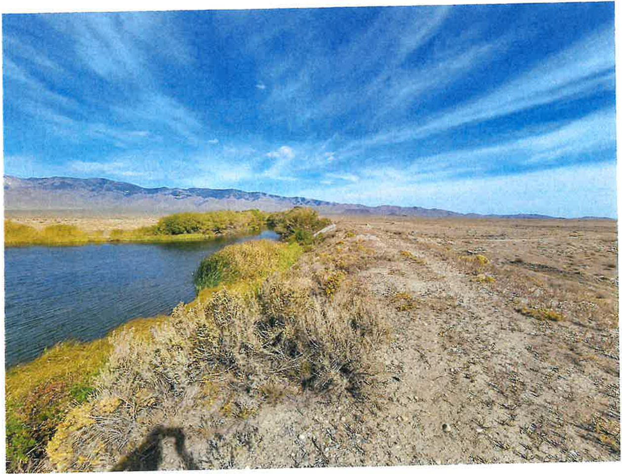
Point of Diversion
