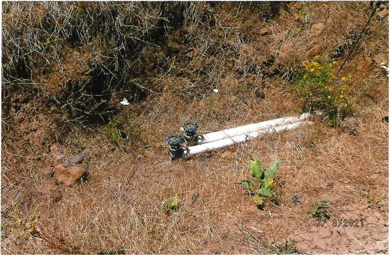
2EA PVC PIPES DAYLIGHT EAST OF GRAVEL ROAD WAY – ALLOW FIRE HOSE CONNECTION TO FILL PORTABLE STOCK TANK(S)
