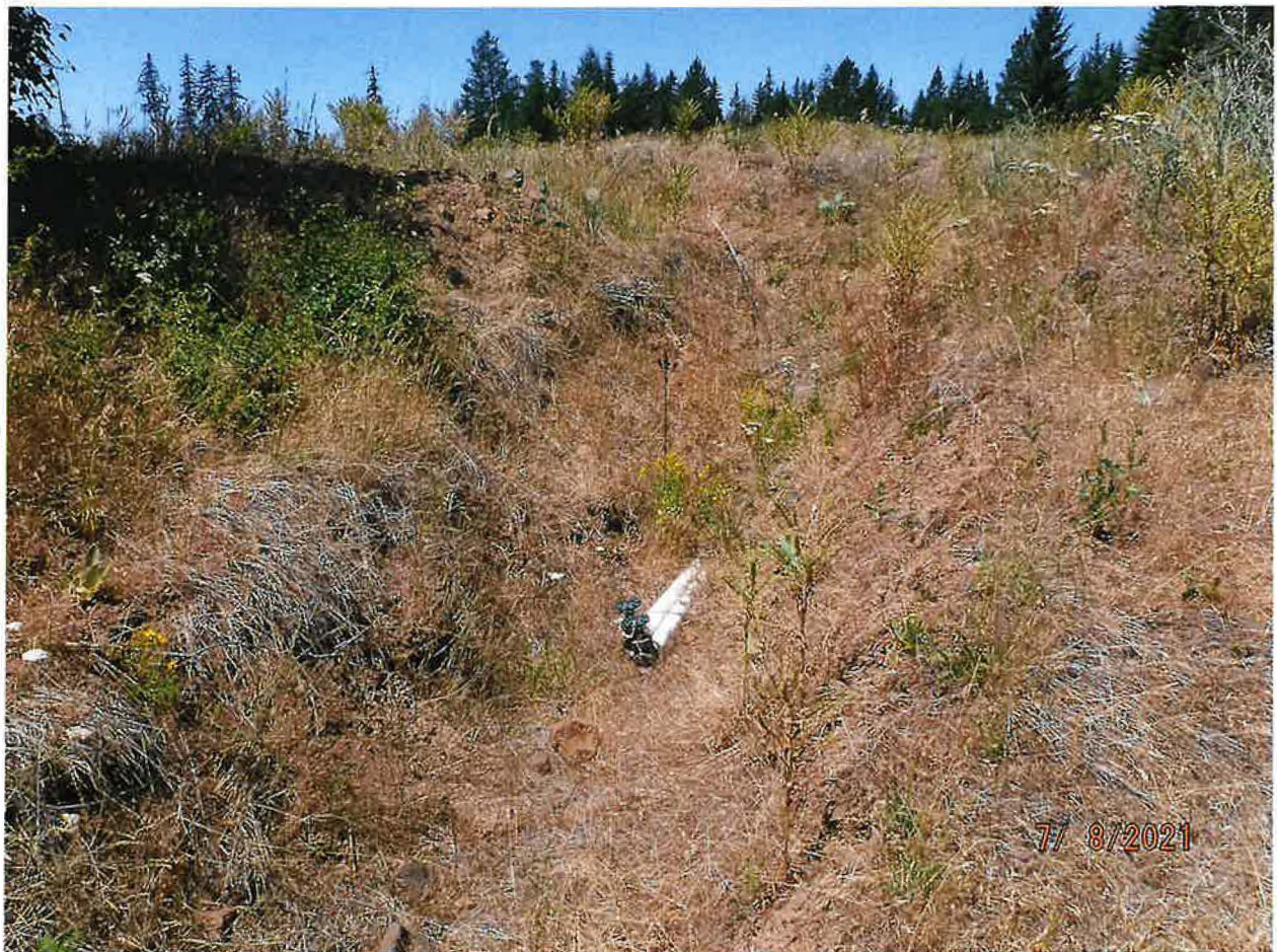
2EA PVC PIPES DAYLIGHT EAST OF GRAVEL ROAD WAY – ALLOW FIRE HOSE CONNECTION TO FILL PORTABLE STOCK TANK(S)
