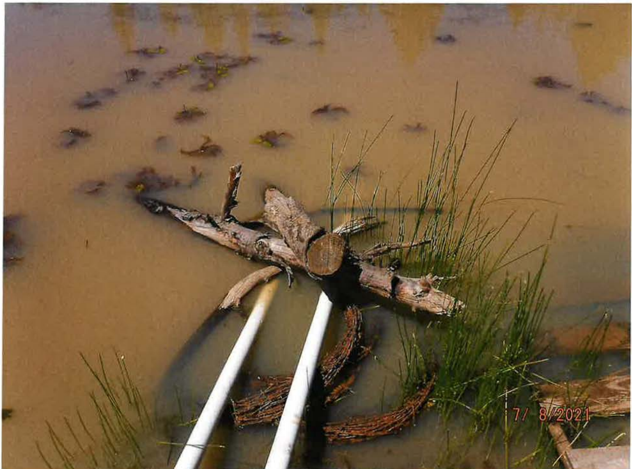
2EA 2 INCH PVC PIPES DRAW WATER FROM POND FOR BENEFICIAL USE(S)
