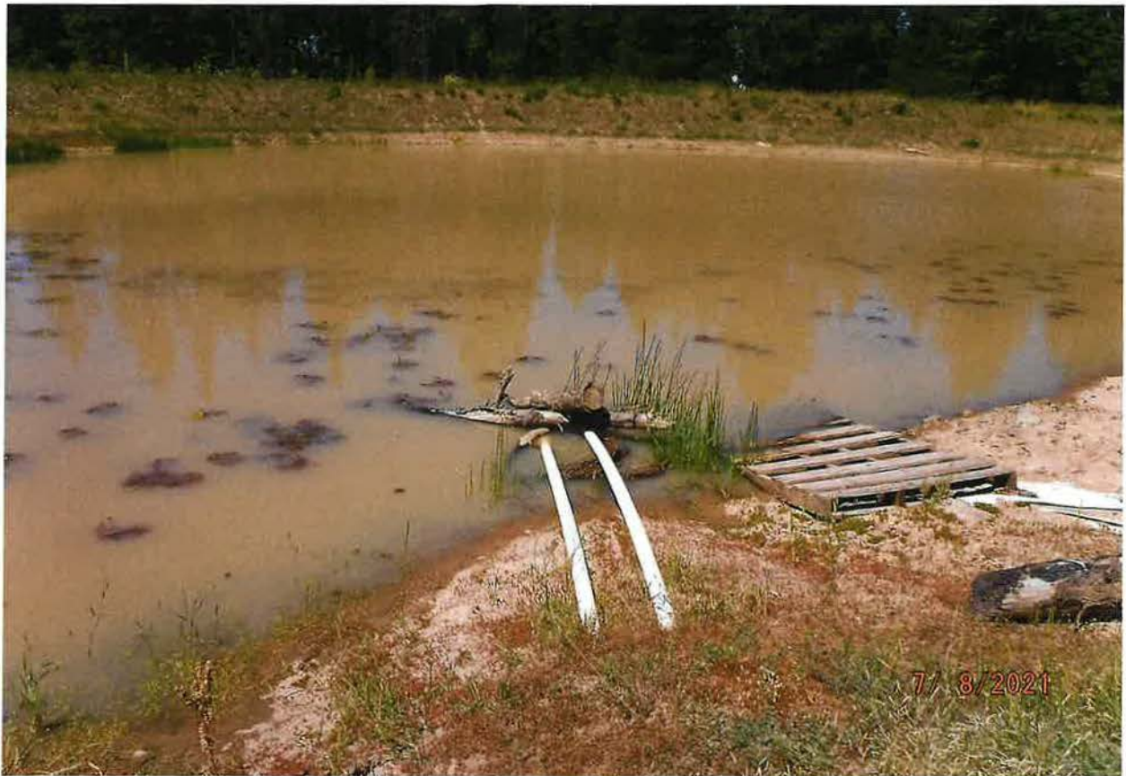
2EA 2 INCH PVC PIPES DRAW WATER FROM POND FOR BENEFICIAL USE(S)
