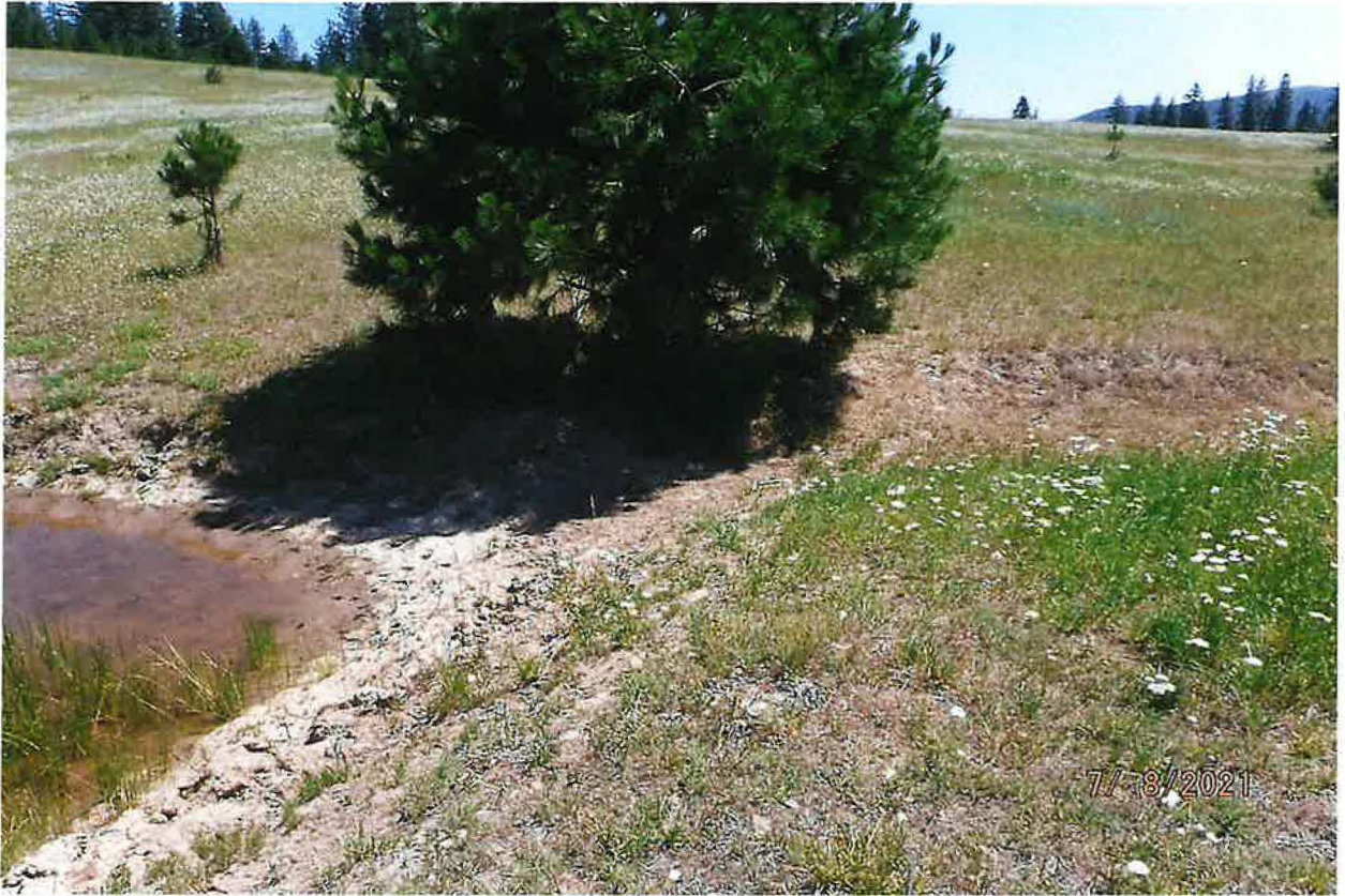
POND 1 OVERFLOW CHANNEL
