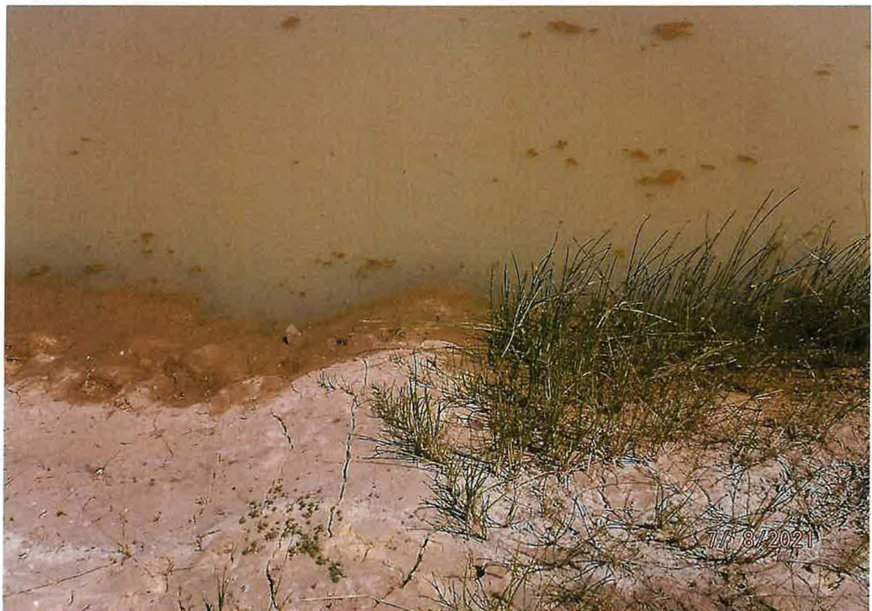
POND 2 FROM STORAGE USE PIPE INSTALLED
