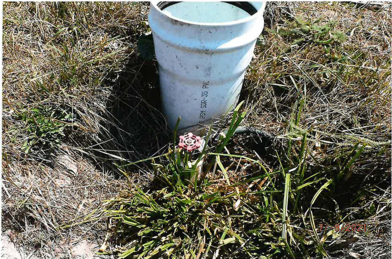
STOCKWATER FROM STORAGE POU – RISER PIPE TO HOSE ENABLES FILLING OF PORTABLE WATER TANKS FOR TROUGHS
