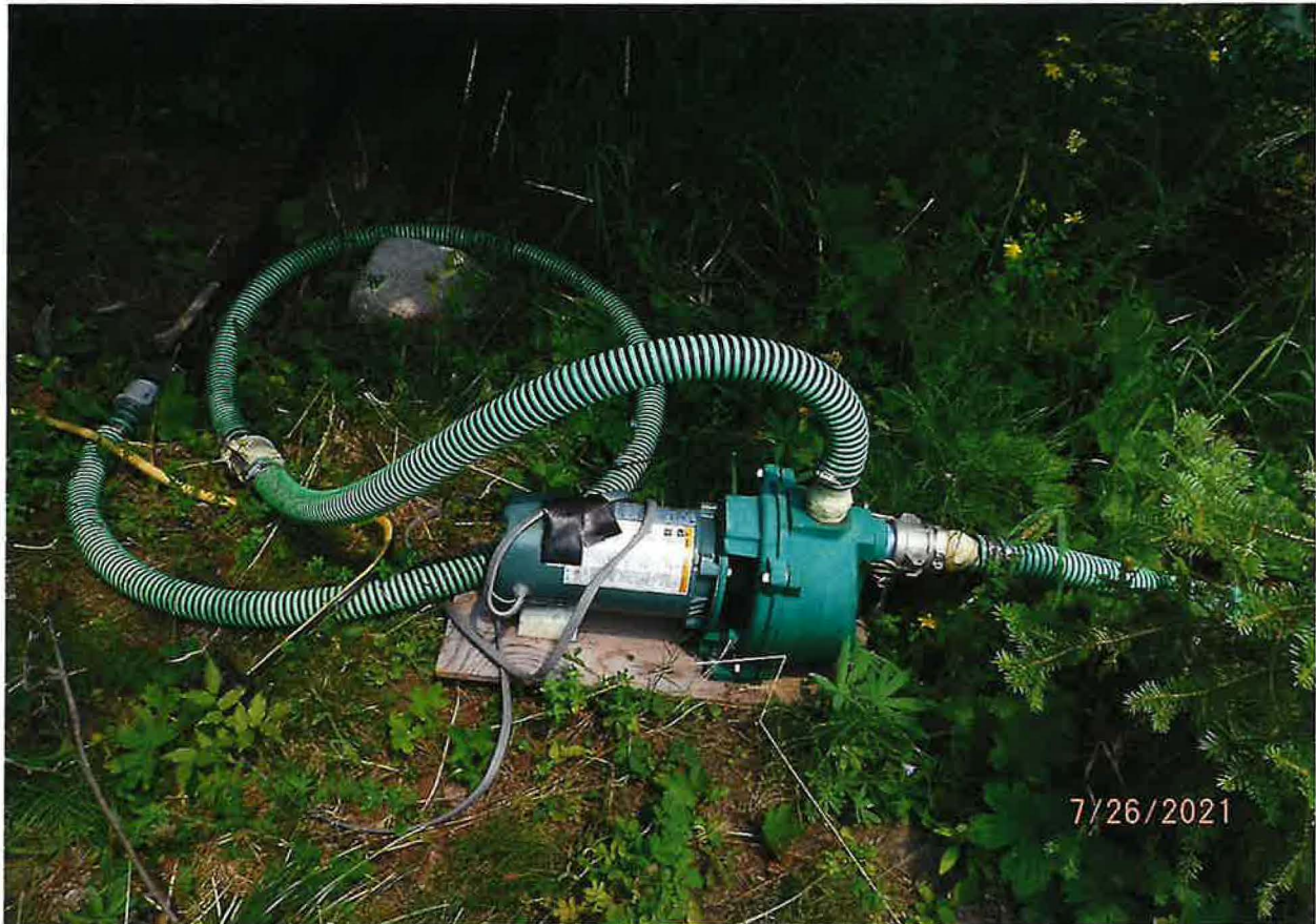
DIVERTING WORKS – SAWYERS PUMP WITH 1 HP PENTEK PUMP MOTOR (SAME POD AS 81-12013)
