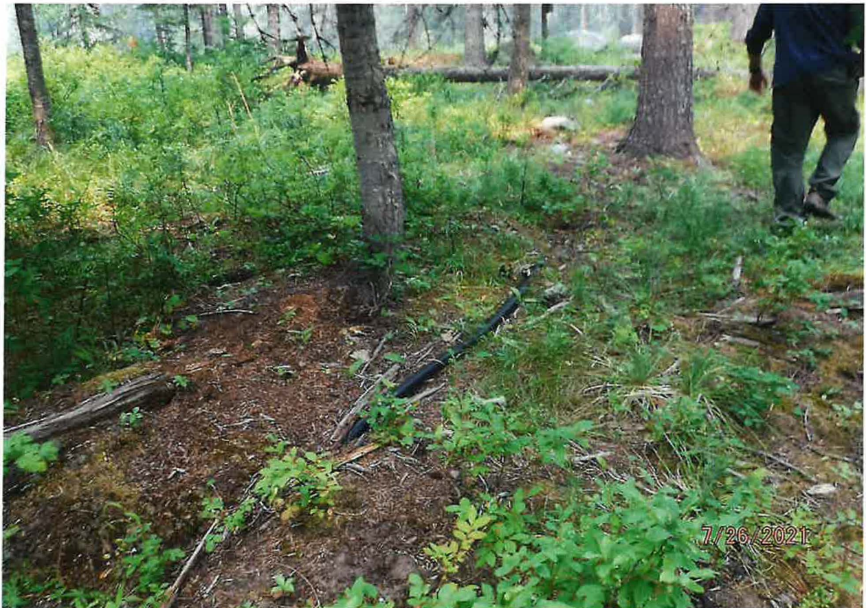
MAIN IRRIGATION POLY PIPE ROUTES THROUGH FORESTED LOT AT IRRIGATION POU
