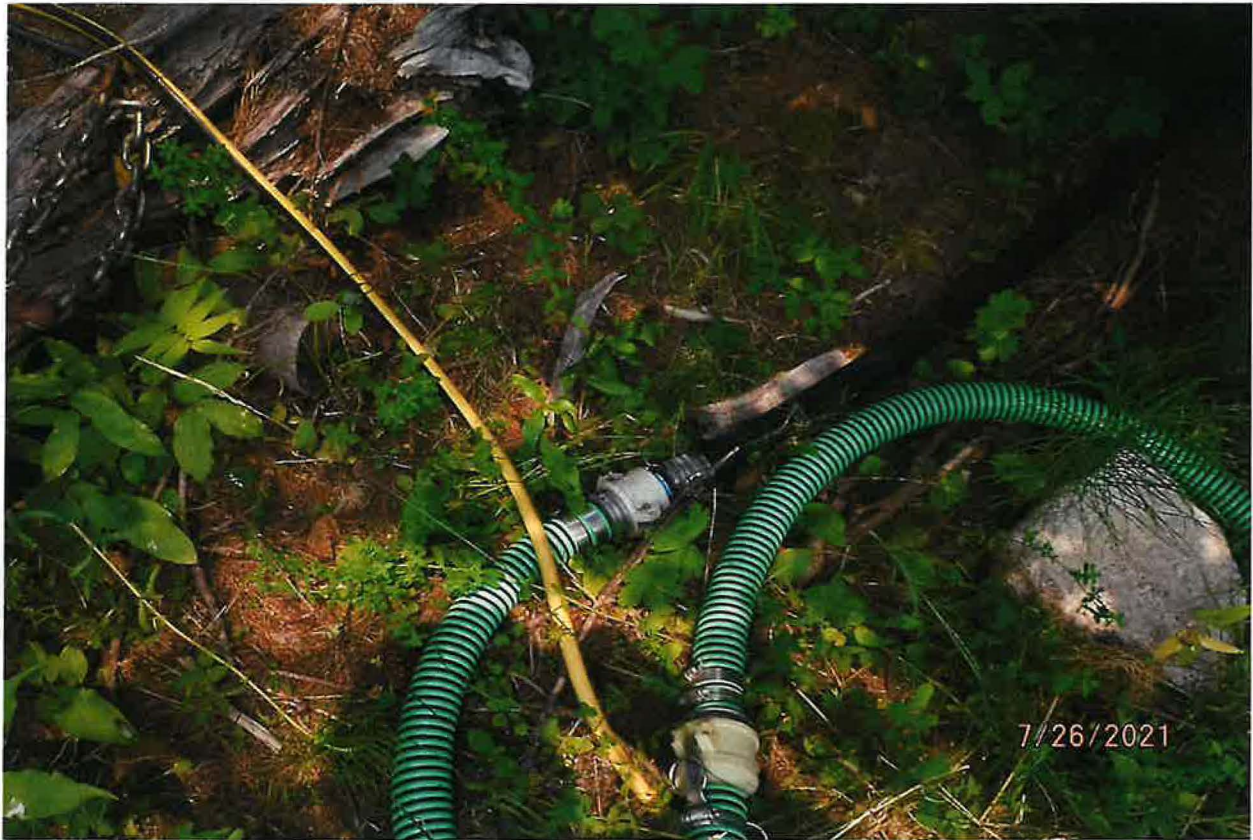
COUPLED FLEX HOSE TO POLY PIPE IRRIGATION MAIN LINE
