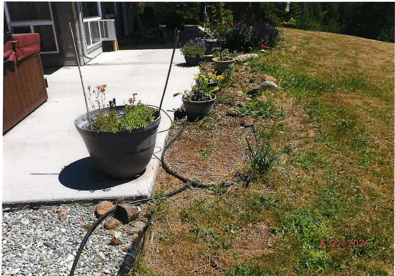
IRRIGATION POU – DRIP LINES ROUTED FOR PLANTS AROUND MAIN HOUSE
