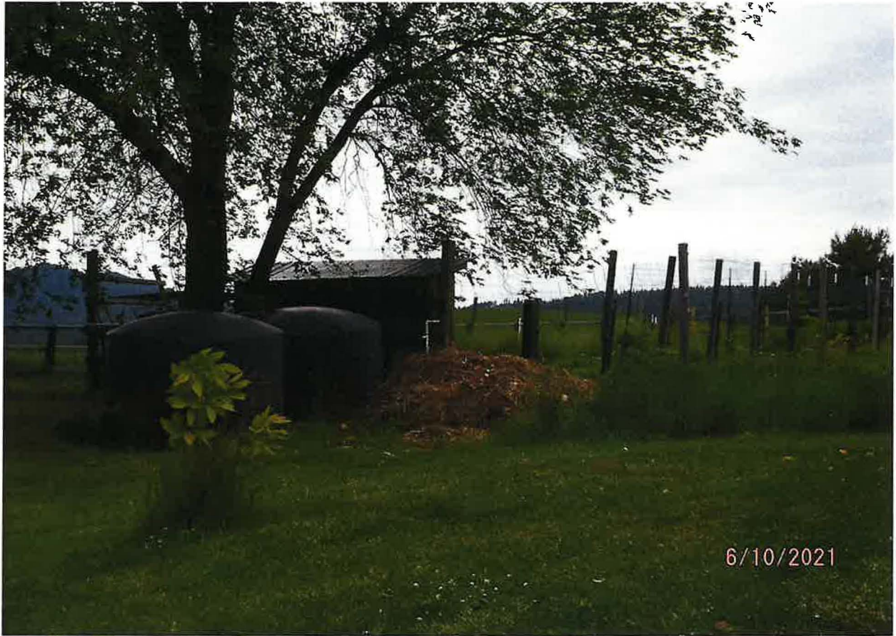
IRRIGATION FROM STORAGE 24 HR IMPOUNDMENT TANKS
