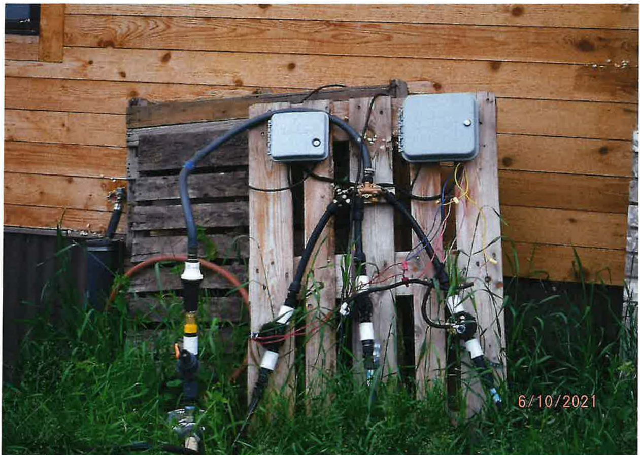
IRRIGATION SYSTEM DIVERTING WORKS
