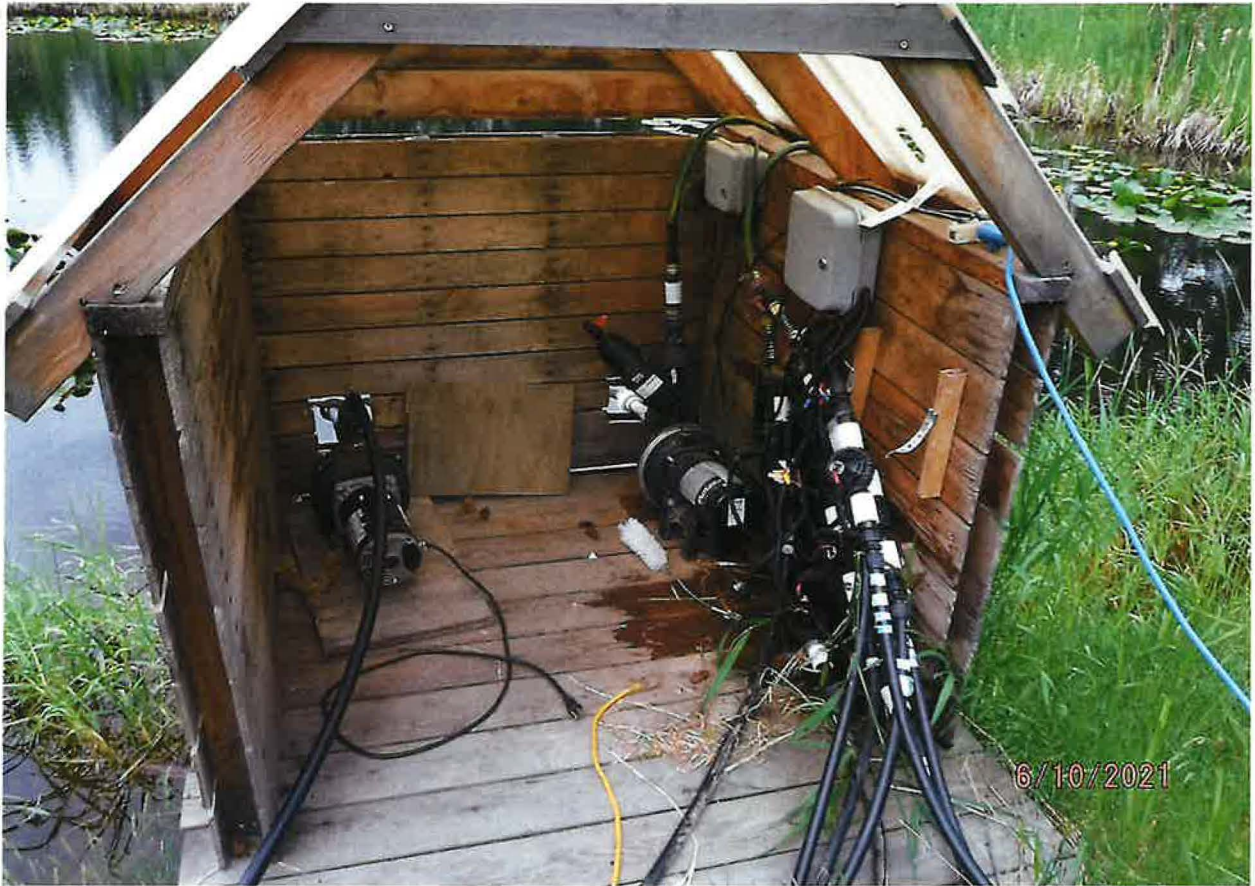
IRRIGATION FROM STORAGE SYSTEM FROM POND 1 – 2EA 1 ½ HP FLOTEC PUMPS
