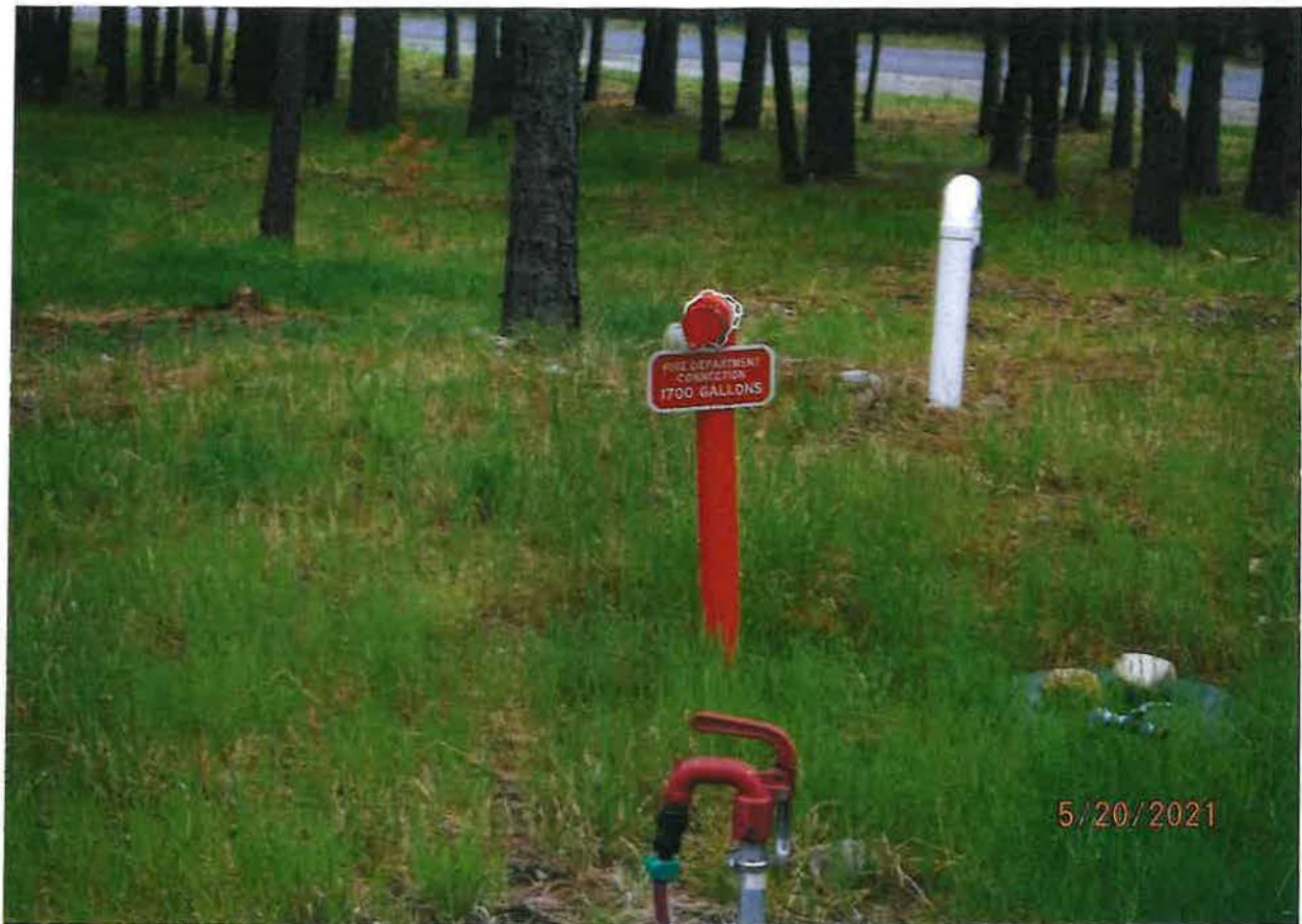
FIRE PROTECTION POU – EXAMPLE FIRE HYDRANT CONNECTION
