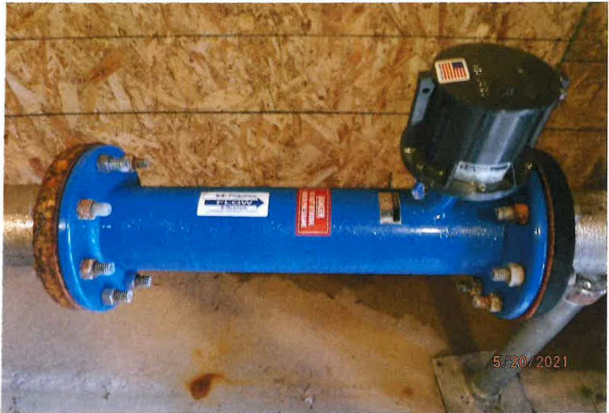
MCCROMETER TOTALIZING FLOW METER – MODEL No. MF104, S/N# 16-12377
