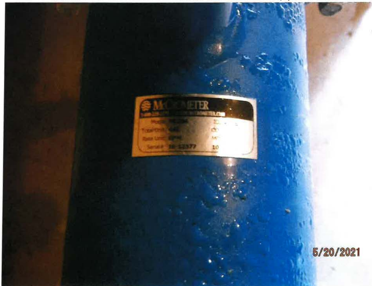
MCCROMETER TOTALIZING FLOW METER – MODEL No. MF104, S/N# 16-12377
